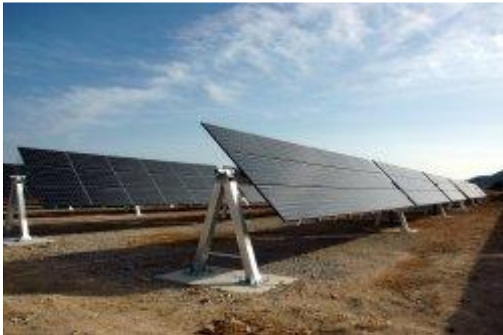
Figure 3. Example of Single Axis Tracking Mount
