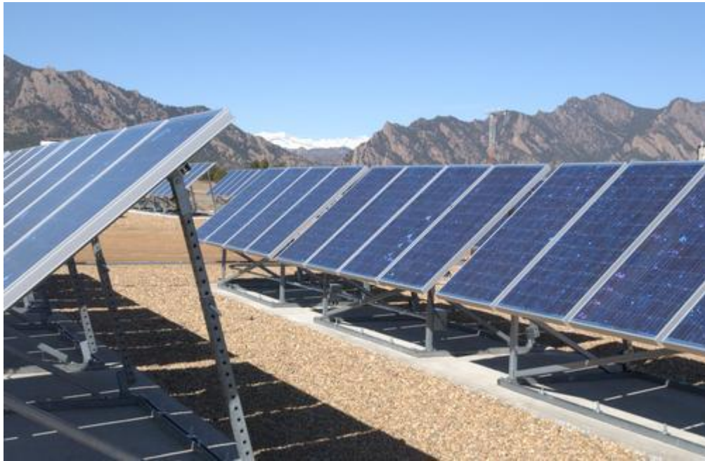
Figure 2. Example of Fixed Tilt Mount
