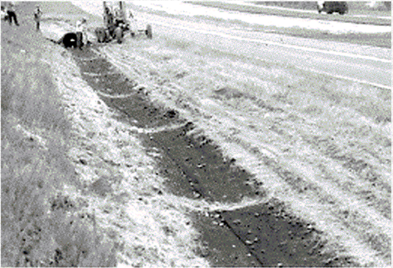
Figure 31. Installed Synthetic Mat Channel Lining
