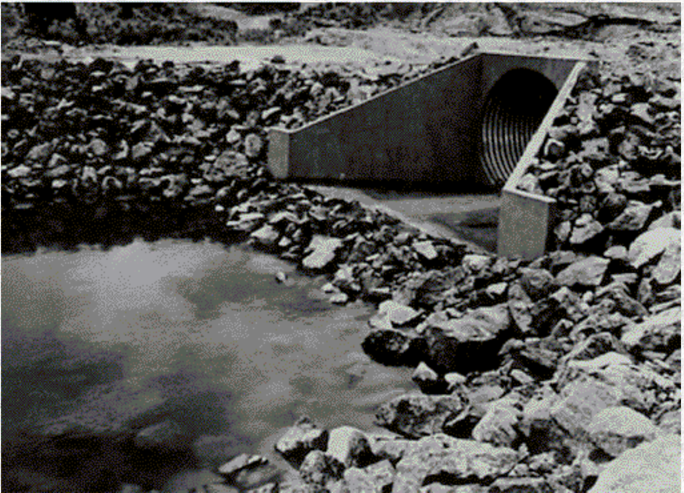
Figure 54. Riprapped Culvert Energy Basin
