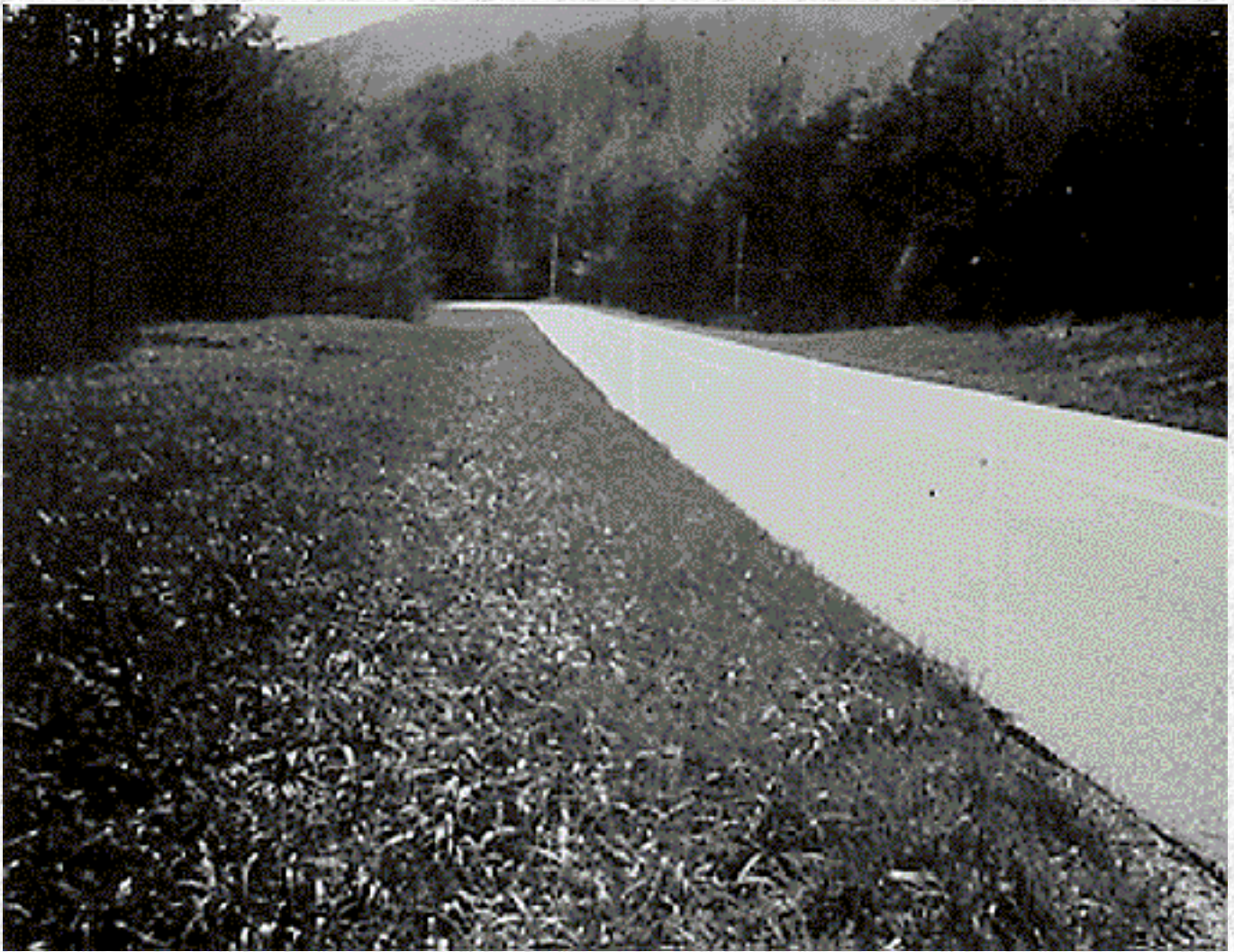
Figure 28. Vegetative Channel Lining
