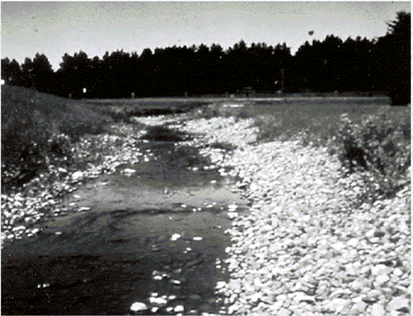
Figure 29. Riprap Channel Lining
