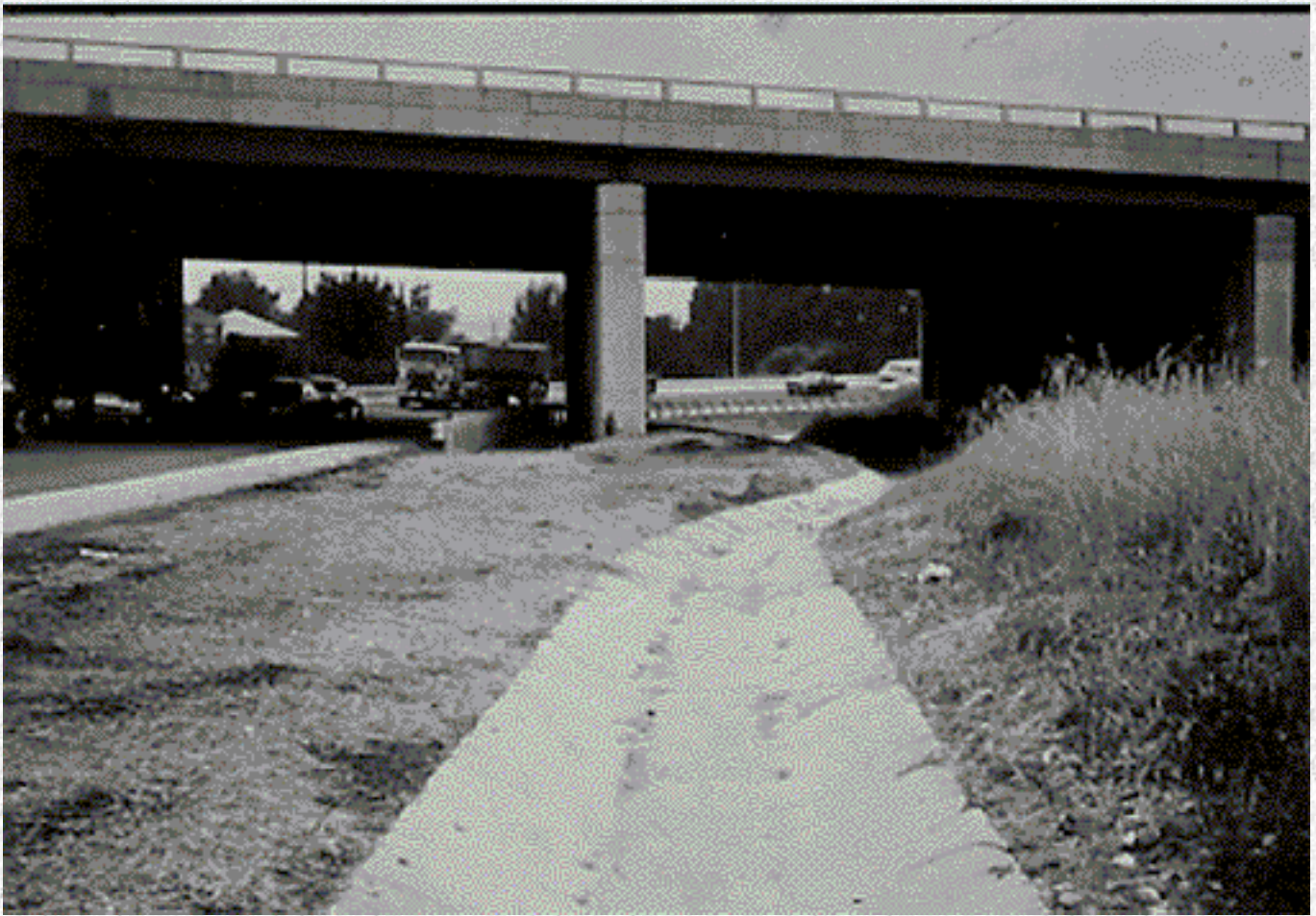
Figure 30. Rigid Channel Concrete Lining
