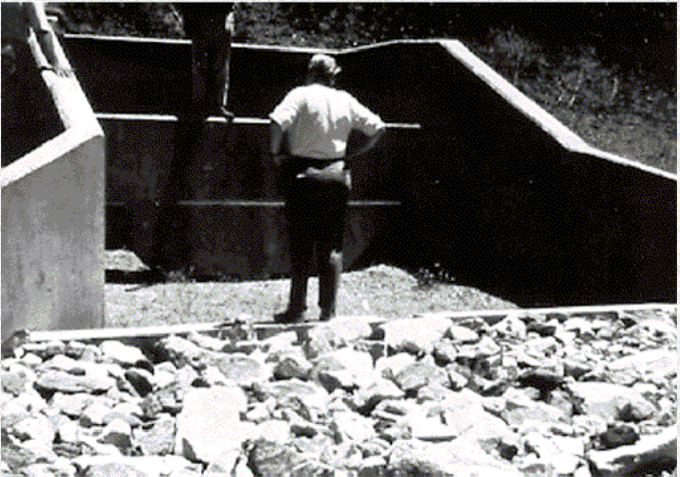
Figure 51b. Baffle-wall Energy Dissipator USBR Type VI
