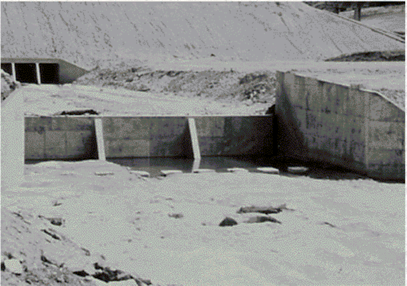
Figure 52. Straight Drop Spillway Stilling Basin
