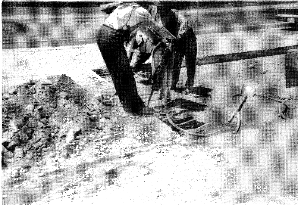
Figure 29. End section removal – using a jackhammer.
