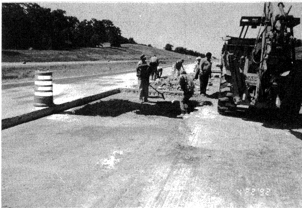
Figure 33. Replacing disturbed subbase with asphaltic concrete.
