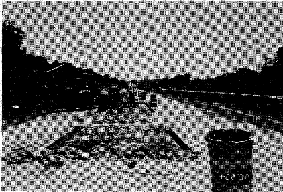
Figure 30. End section removal process.
