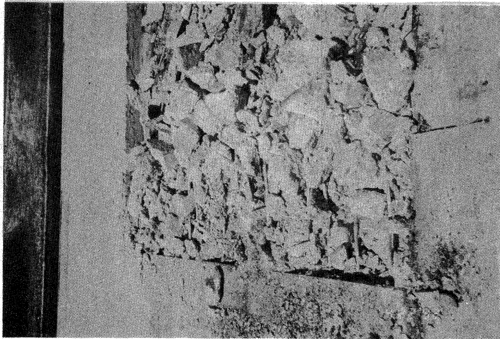
Figure 31. End section removal - close-up view.
