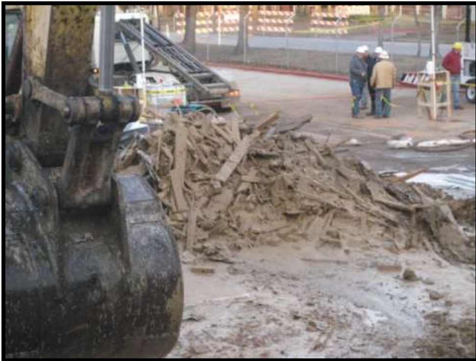
Figure 5-40. Nearing the end of debris removal.
