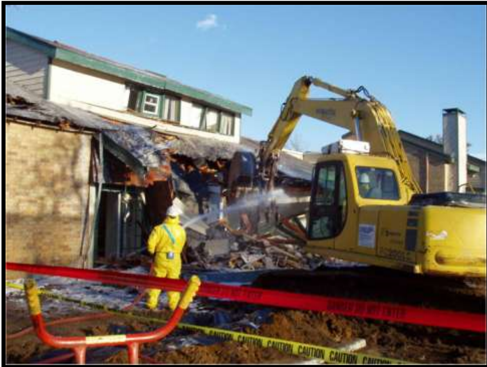
Figure 5-34. More demolition progress.
