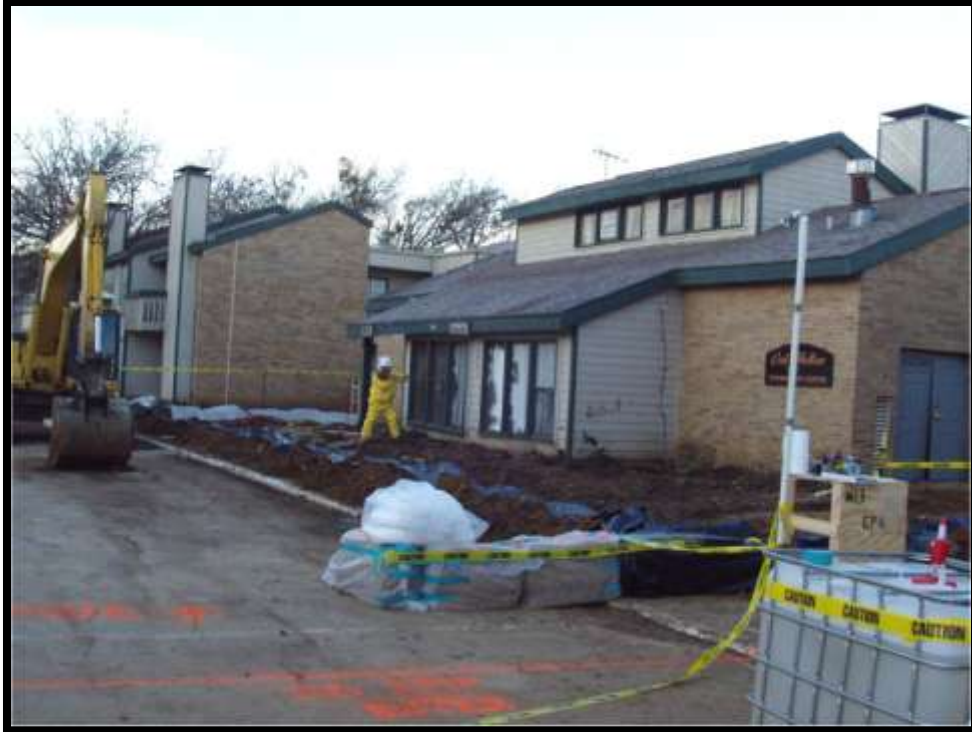
Figure 5-26. Preparing for wetting the day of the demolition (knocking out windows).
