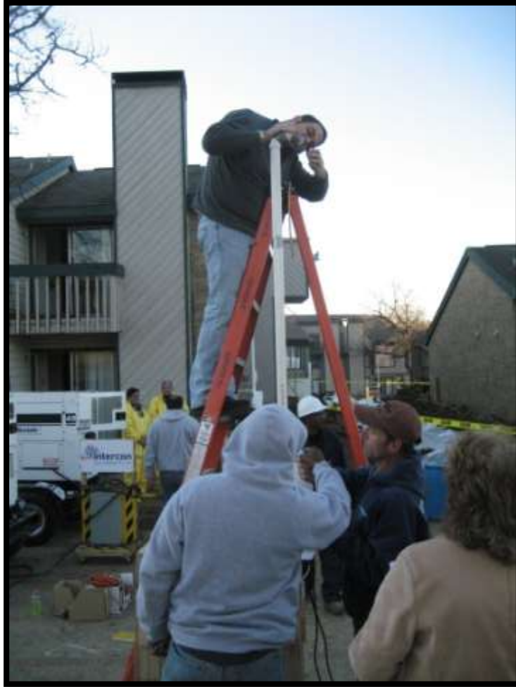
Figure 5-17. Installing filter cartridges on sampler arrays.
