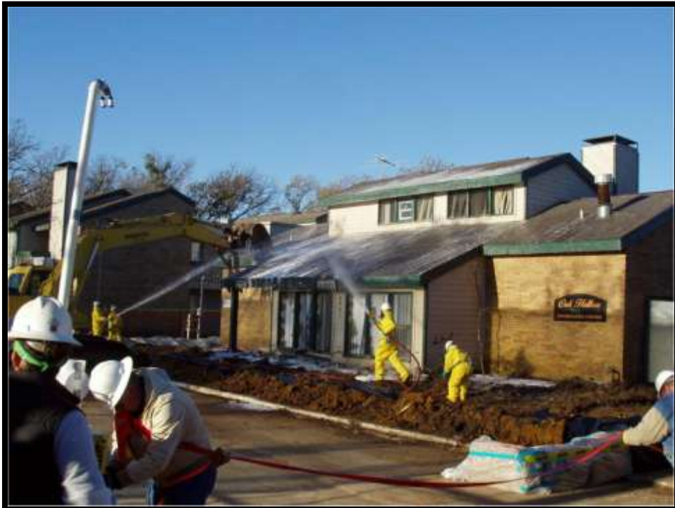
Figure 5-29. Wetting the building before the demolition.
