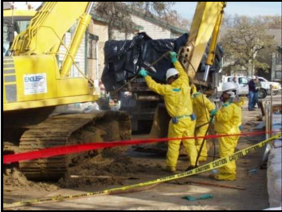
Figure 5-52. Cleaning the track hoe.
