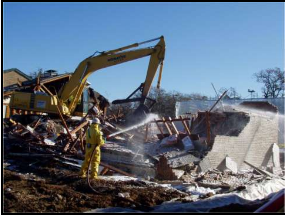
Figure 5-37. More demolition progress.
