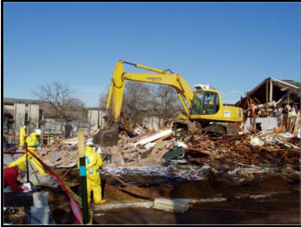
Figure 5-39. More demolition progress.
