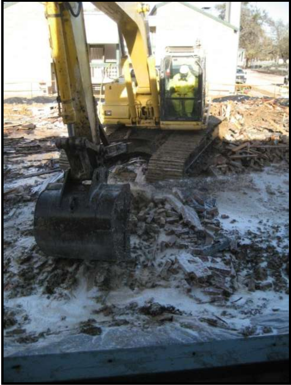
Figure 5-41. Final debris removal.
