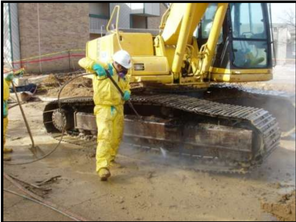
Figure 5-53. Cleaning the track-hoe.
