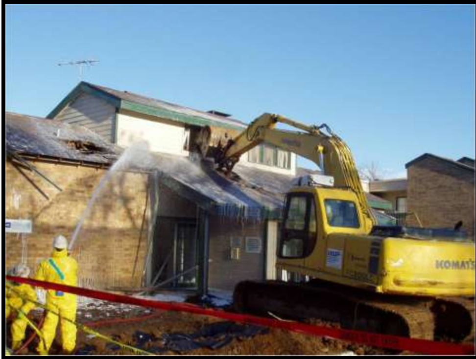
Figure 5-33. More demolition progress.
