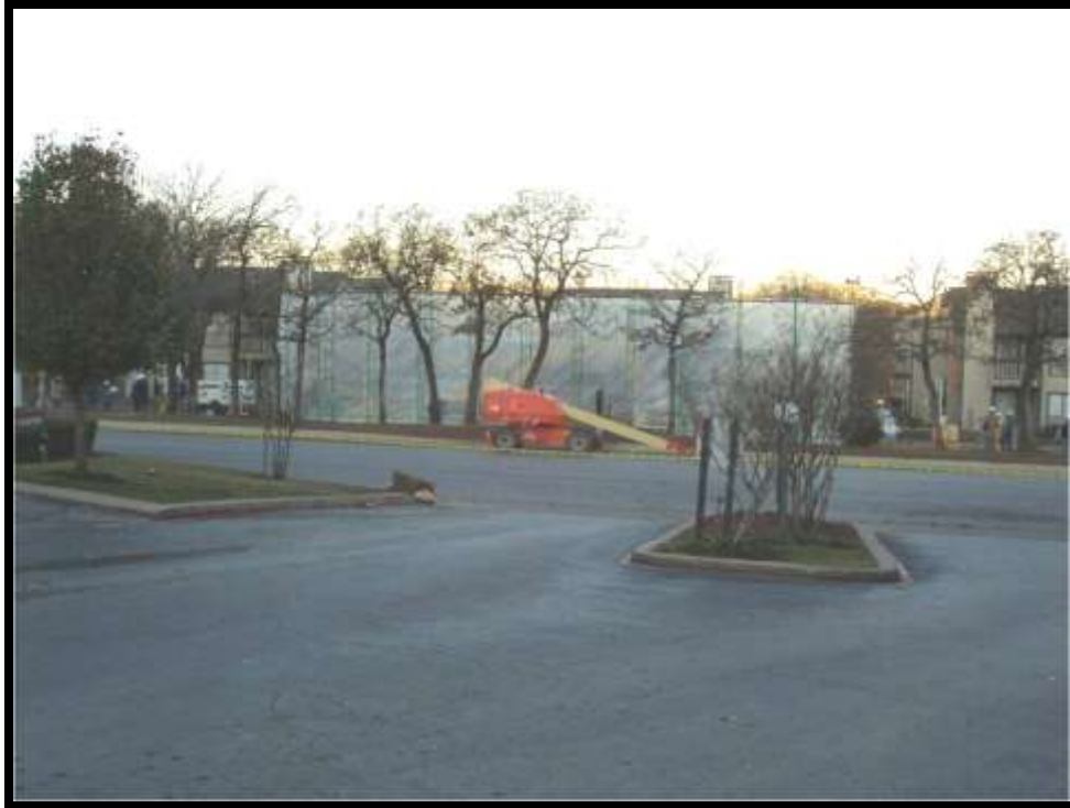
Figure 4-8. Barrier wall as seen from the entrance to occupied apartment complex.
