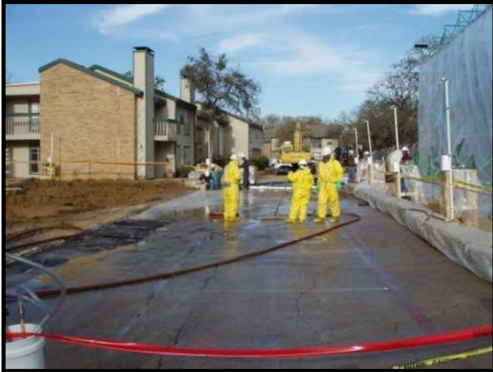
Figure 5-56. Driveway cleaning is almost finished.
