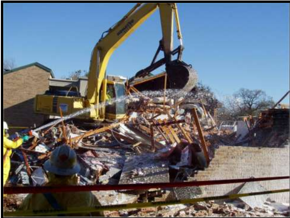
Figure 5-38. More demolition progress.
