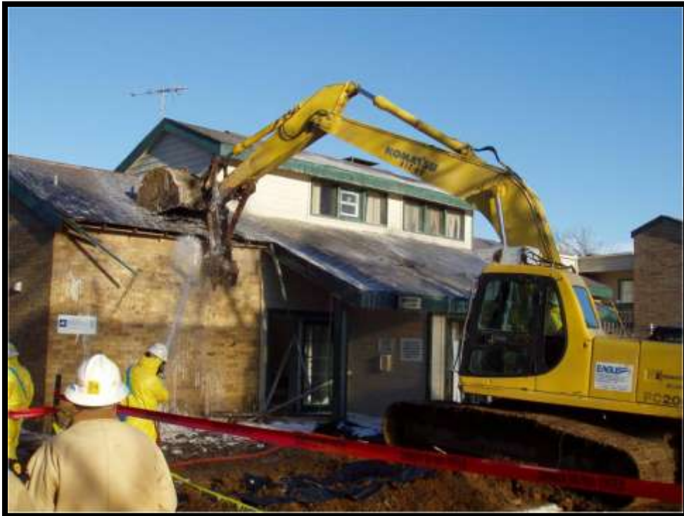
Figure 5-32. Making holes in the roof to the increase wetting.
