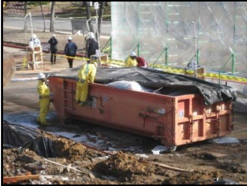
Figure 5-46. Covering the burrito wrap to prepare the roll-off for removal.
