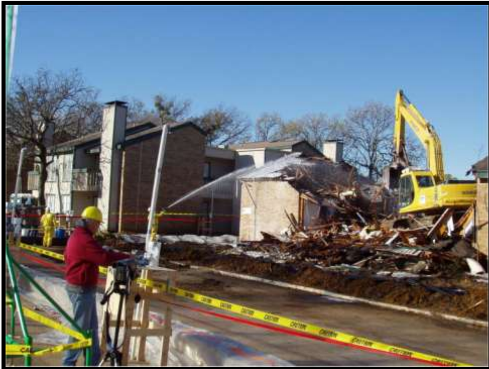
Figure 5-36. More demolition progress.
