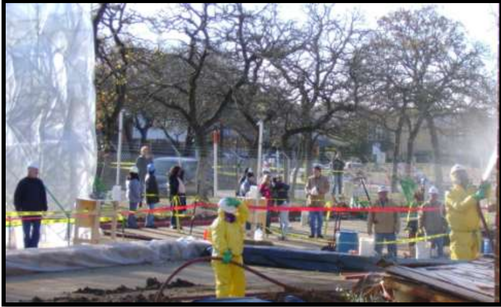
Figure 4-11. Television coverage of the demolition.
