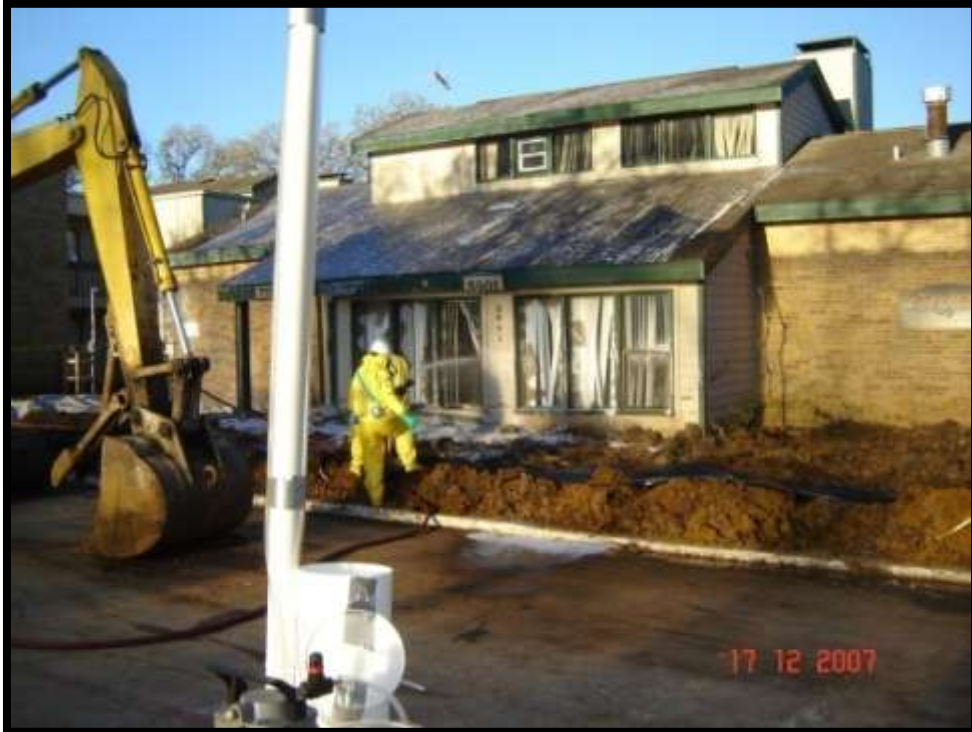
Figure 5-27. Wetting the interior.
