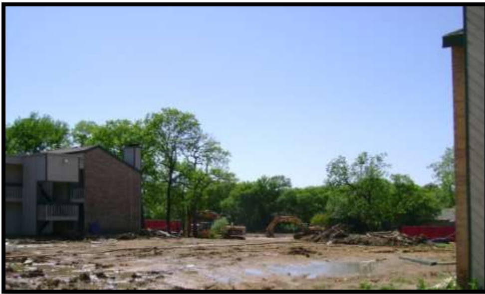
Figure 5-59. Site later after slab removal.
