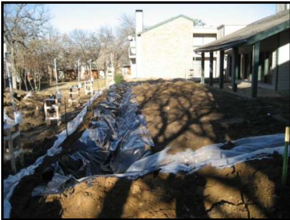
Figure 5-14. Plastic-lined ditches in the rear of the building.
