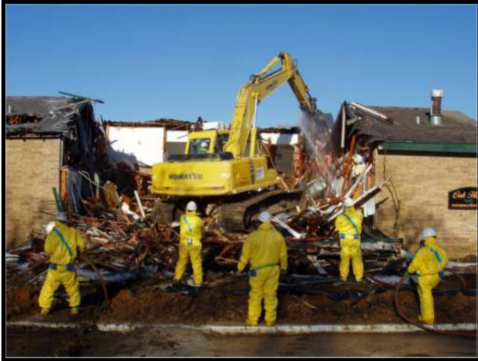
Figure 5-35. More demolition progress.
