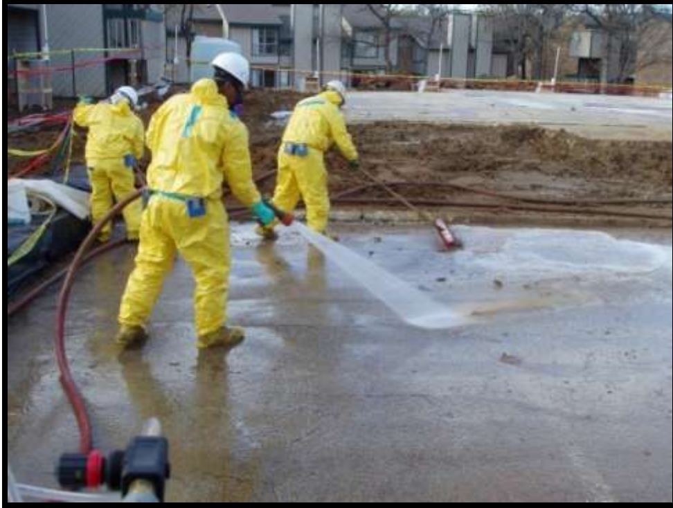
Figure 5-54. Cleaning the driveway.
