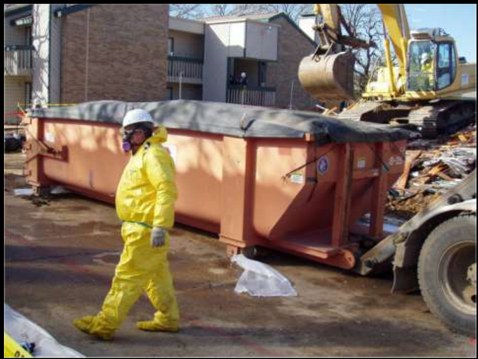
Figure 5-47. Loading the covered roll-off onto the truck.
