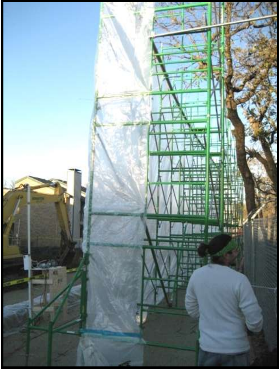
Figure 4-7. Scaffolding and plastic covering for the barrier wall.
