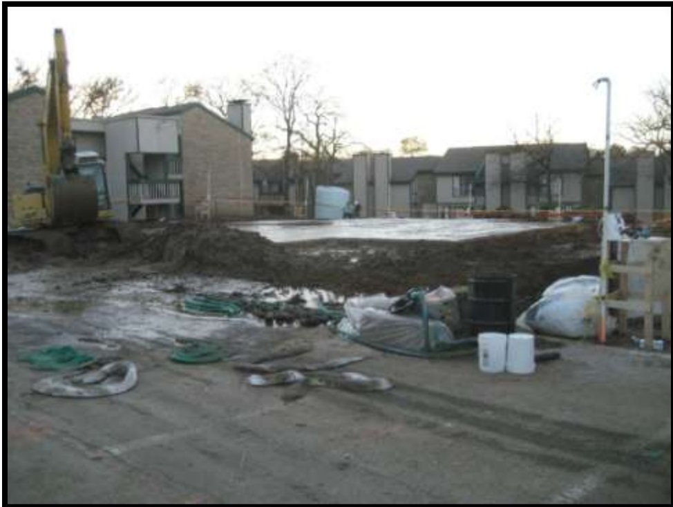
Figure 5-51. Nearing completion except for driveway cleaning.
