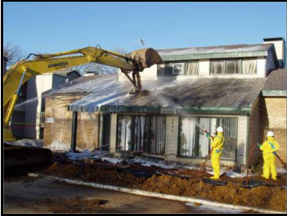
Figure 5-31. Starting the demolition.
