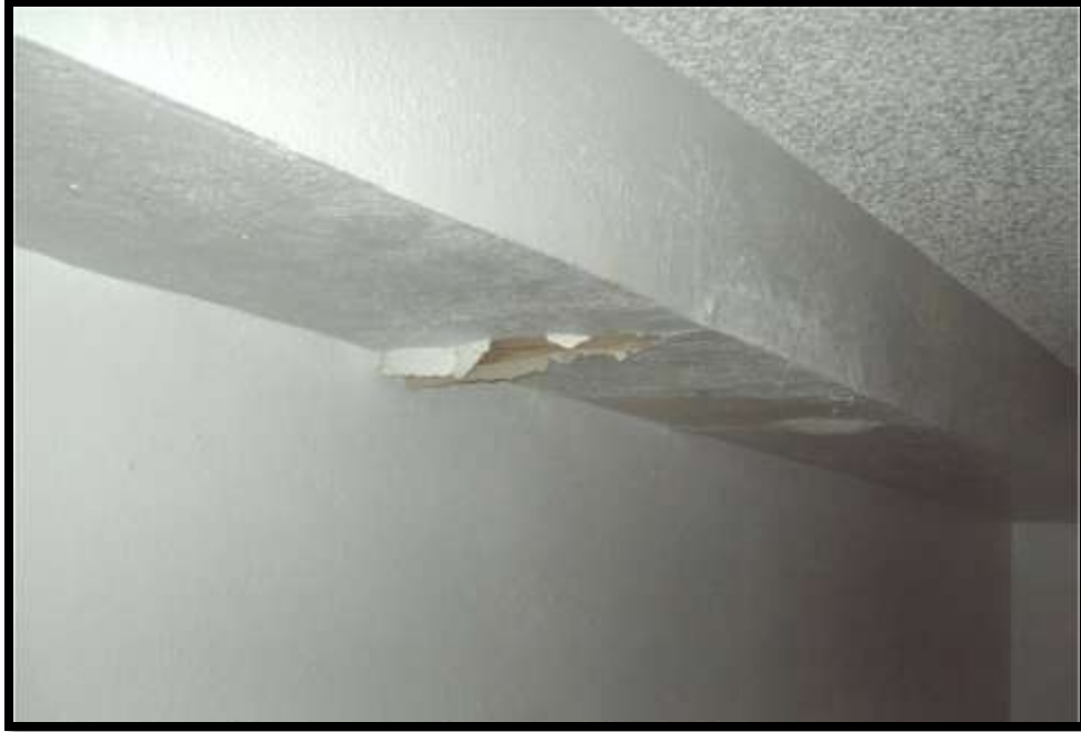
Figure 5-24. More delamination.
