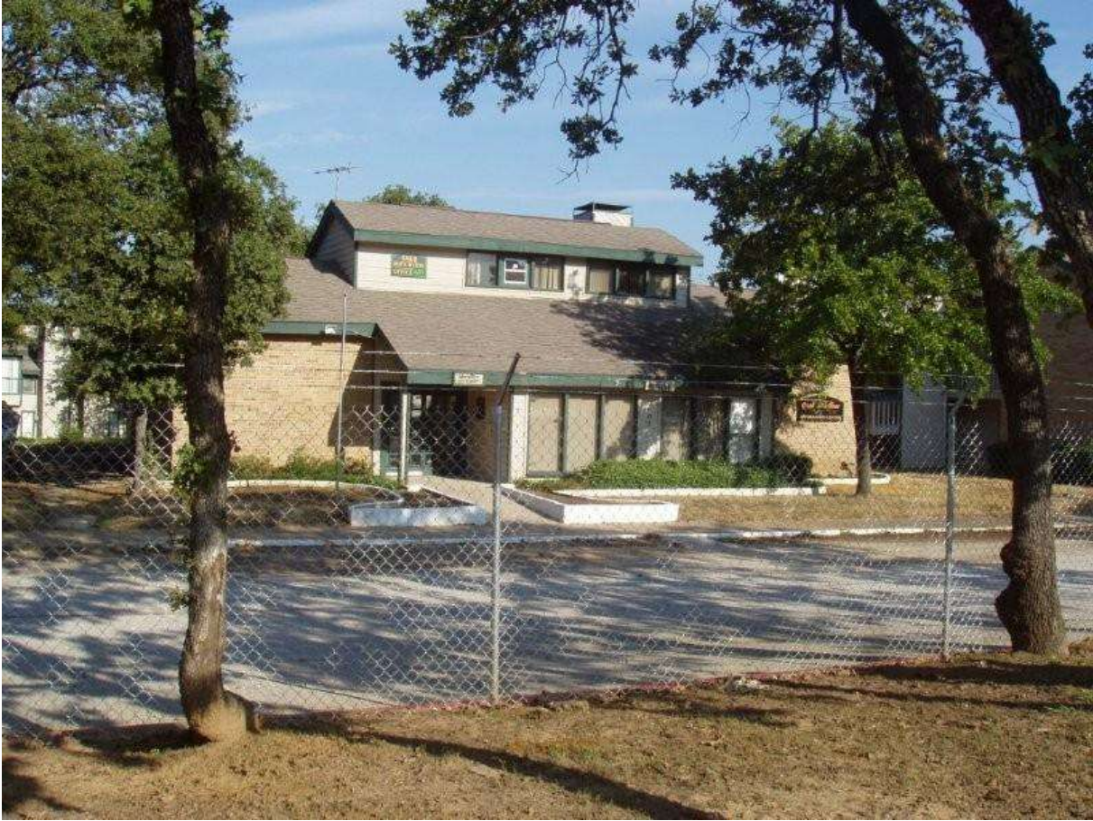
Figure 4-1. Oak Hollow apartment complex office building.
