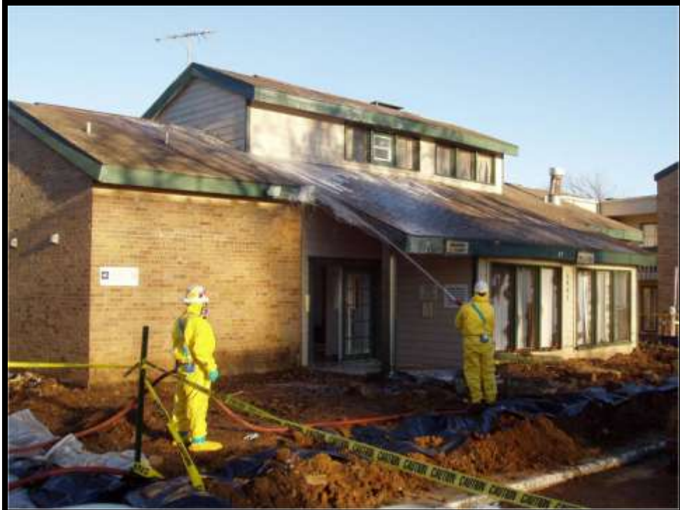
Figure 5-28. Starting to wet the exterior on the morning of the demolition.
