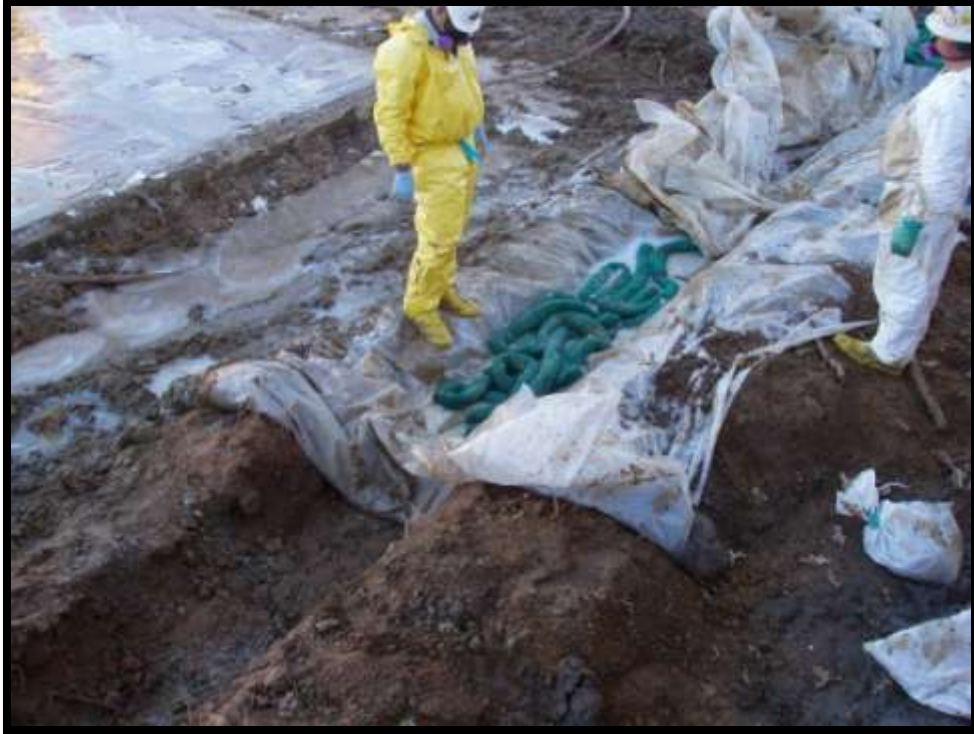
Figure 5-50. Removing the ditch liners.
