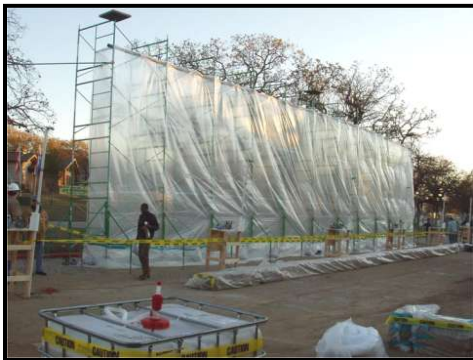
Figure 4-6. Barrier wall looking toward Boca Raton Boulevard.
