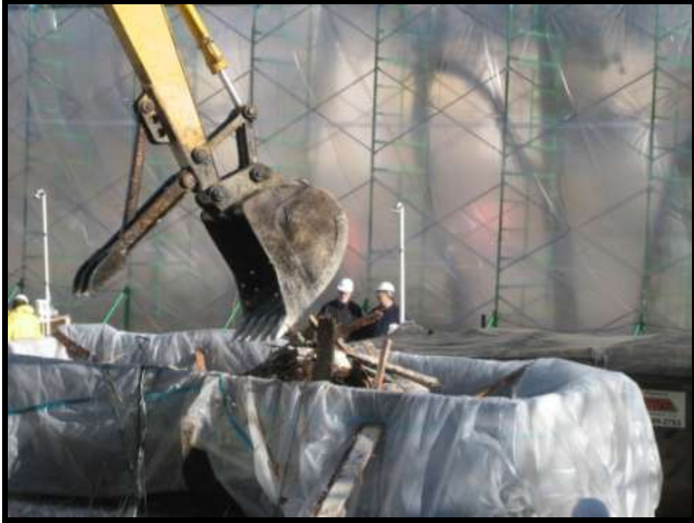
Figure 5-44. Loading a lined roll-off.
