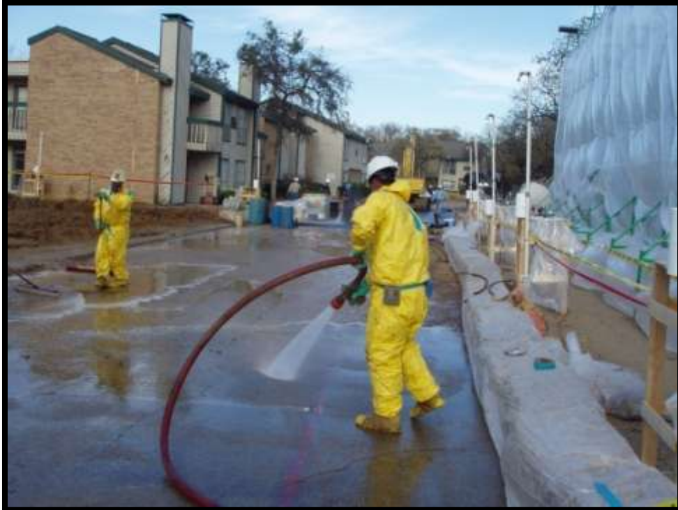
Figure 5-55. Cleaning the driveway.
