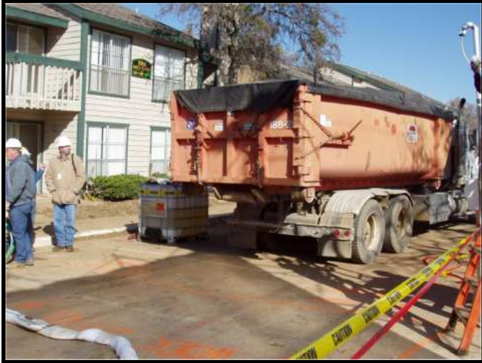
Figure 5-48. Removing the roll-off from the site.
