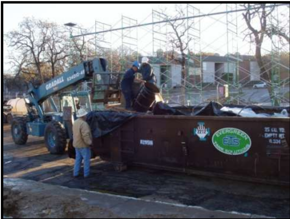
Figure 5-57. Completing final load for landfill.
