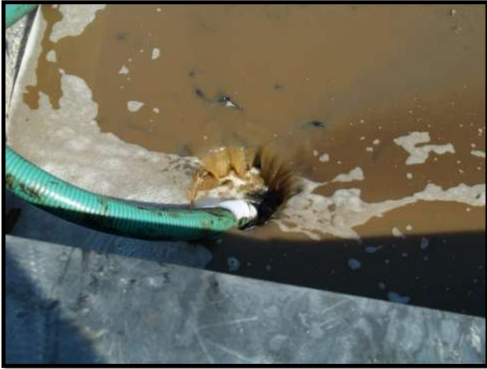
Figure 5-9. Pooled surface water collection sump.
