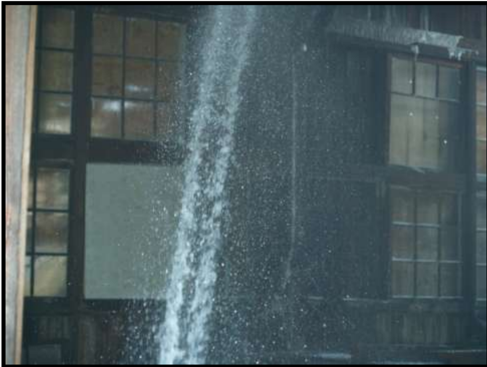
Figure 5-27. Wetting the interior the morning of the demolition.
