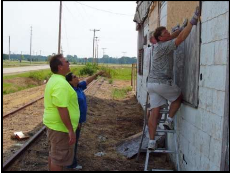
Figure 4-8. Boarding the openings to prepare for applying additional transite.
