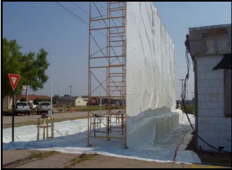
Figure 4-15. The barrier wall in place at the rear of the building.
