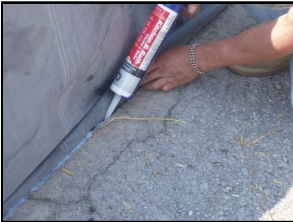
Figure 5-6. Sealing barrier into kerf in pavement.
