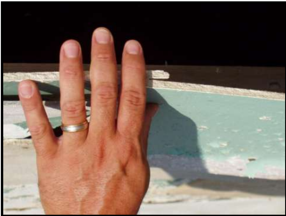
Figure 4-11. Close-up of the added transite from Fort Hood.
