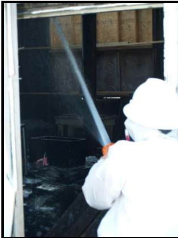
Figure 5-25. Wetting the interior the morning of the demolition.
