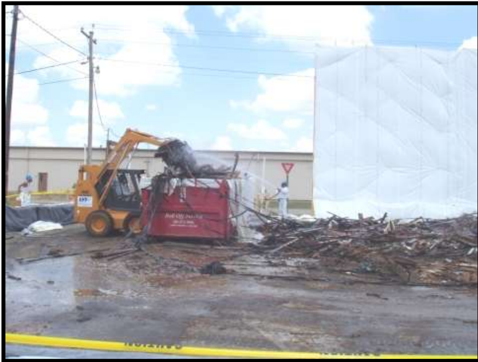
Figure 5-38. Load-out the AACM demolition debris (note Velcro).
