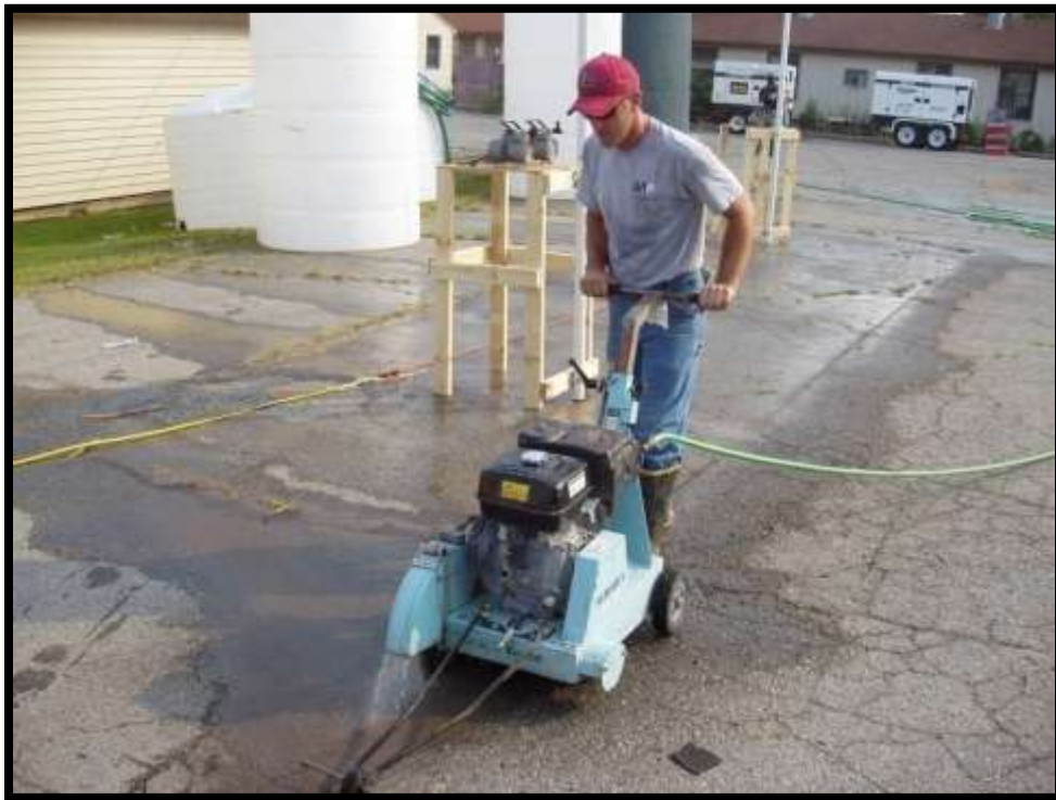
Figure 5-4. Preparing kerf in asphalt to construct barrier.
