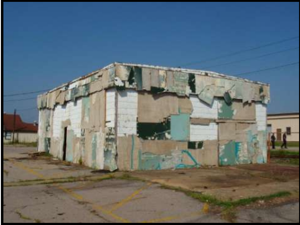
Figure 4-10. End view of the building after the extra transite addition.
