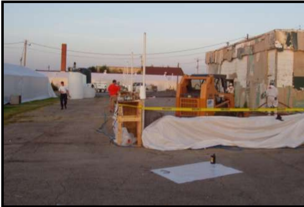
Figure 5-3. Site preparation including covering adjacent buildings.
