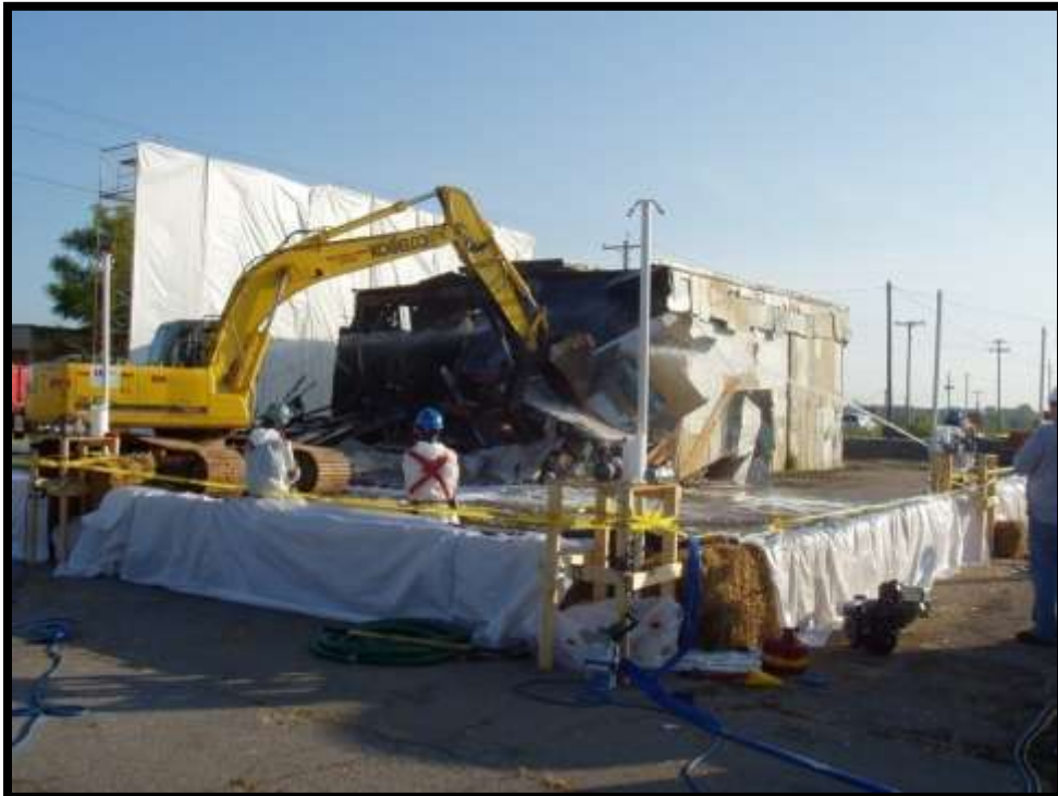
Figure 5-32. Demolition barely underway.
