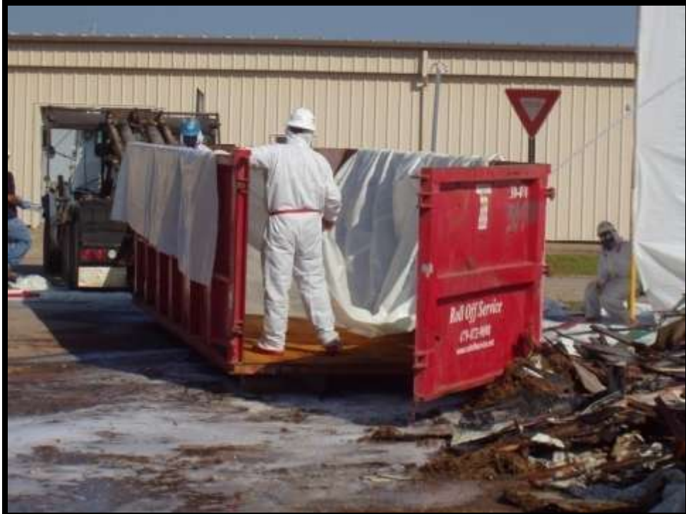
Figure 5-29. Double-lining the roll-offs for hauling of the AACM debris.
