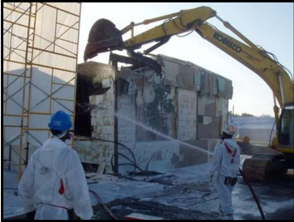
Figure 5-31. Progressing with the AACM demolition.
