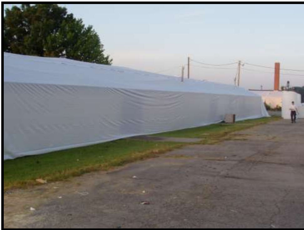
Figure 4-22. Adjacent buildings were covered.
