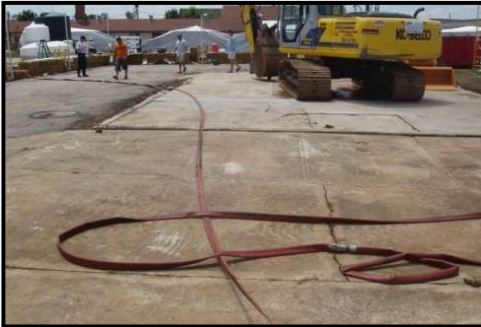
Figure 5-47. Nearing the completion of the ACM demolition.
