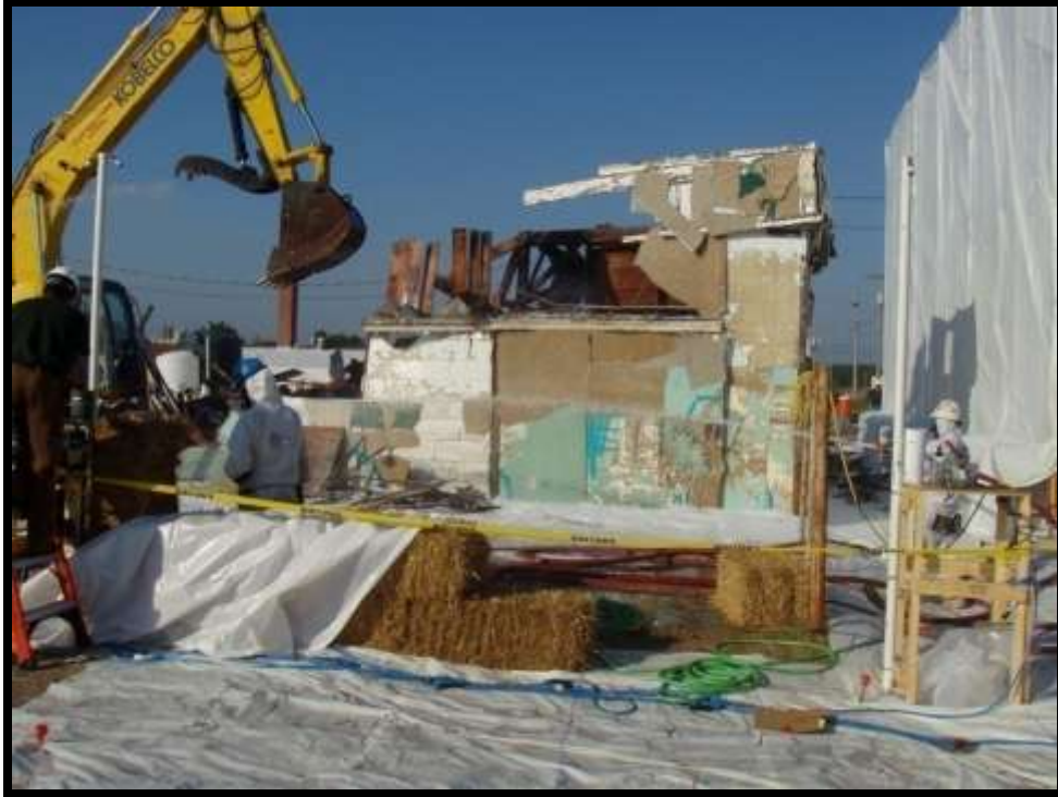
Figure 5-33. Transite building about one-third demolished.
