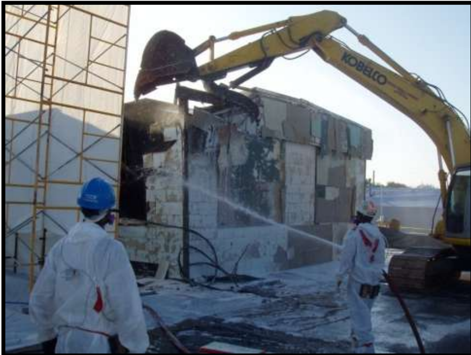
Figure 5-30. Starting the AACM demolition.
