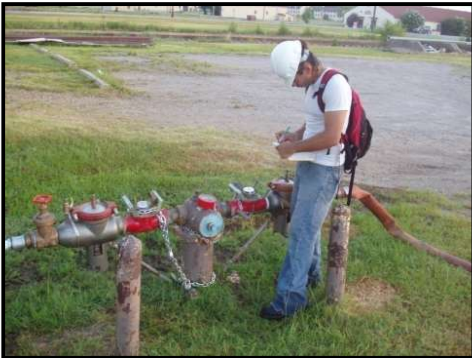
Figure 5-20. Documenting water usage.
