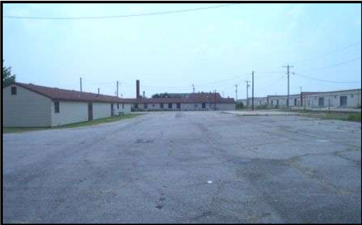
Figure 5-49. After completion of the AACM demolition.
