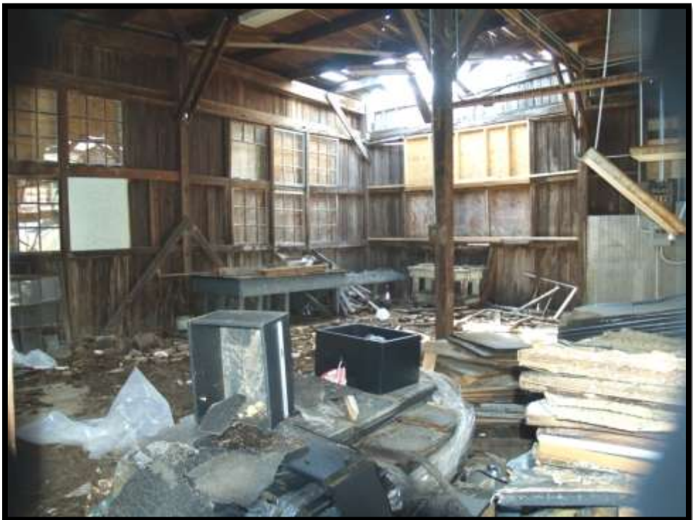
Figure 4-6. Interior view of transite building showing stockpiled materials.
