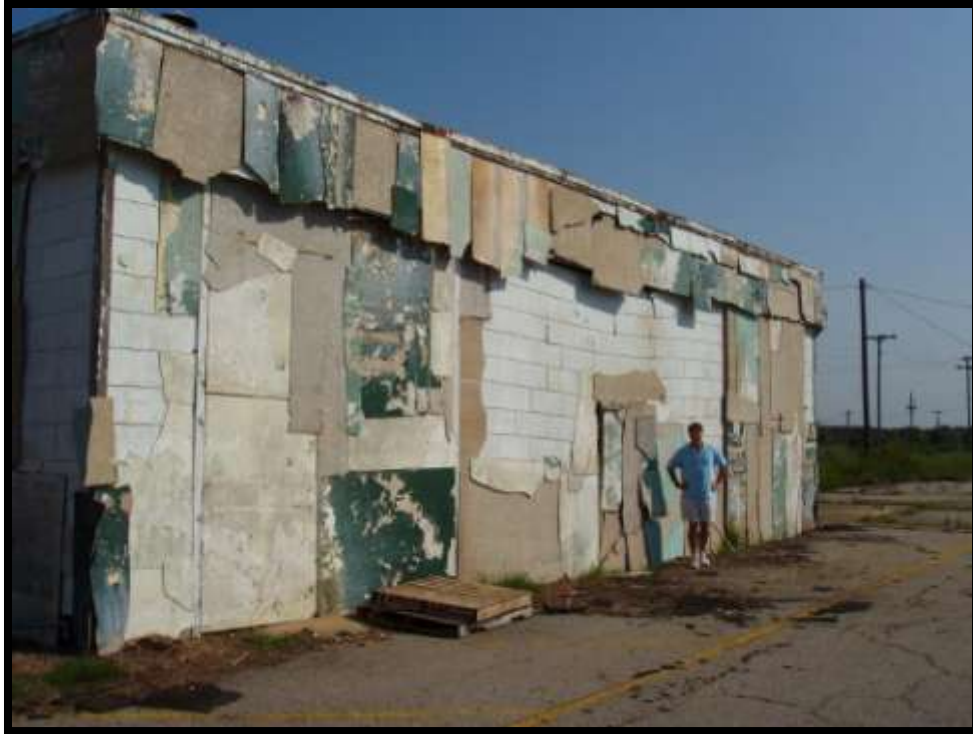
Figure 4-12. Front view of the building after the extra transite addition.
