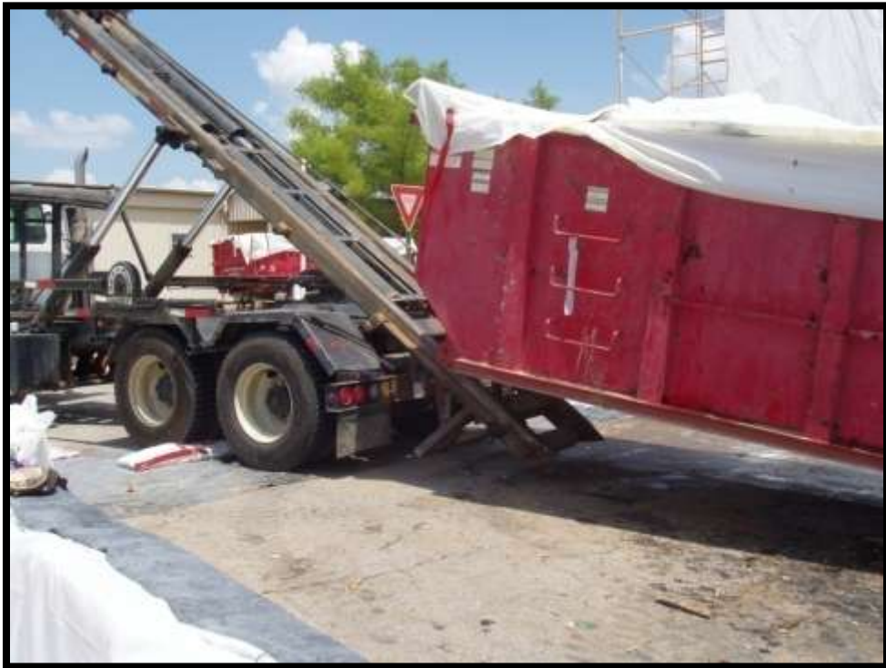
Figure 5-42. Removing the roll-off from the containment area.
