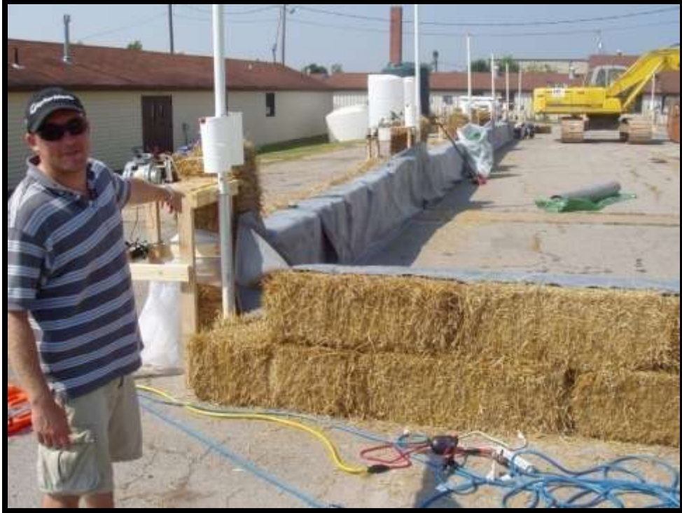
Figure 5-7. Finished barrier to prevent water runoff from site.
