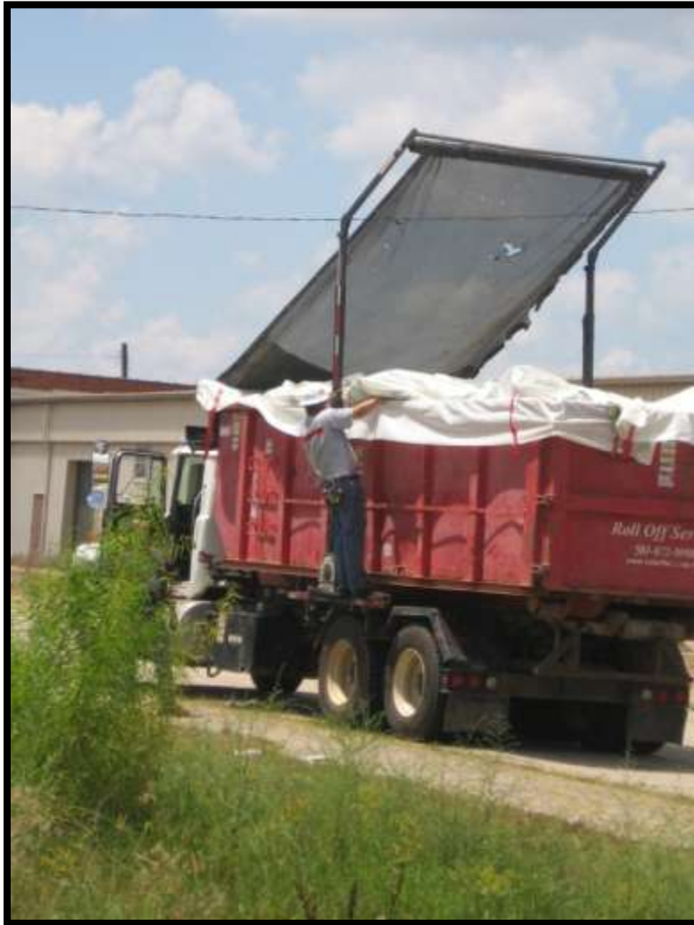
Figure 5-43. Additional covering before the trip to the landfill.
