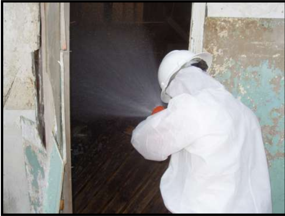
Figure 5-26. Wetting the interior the morning of the demolition.
