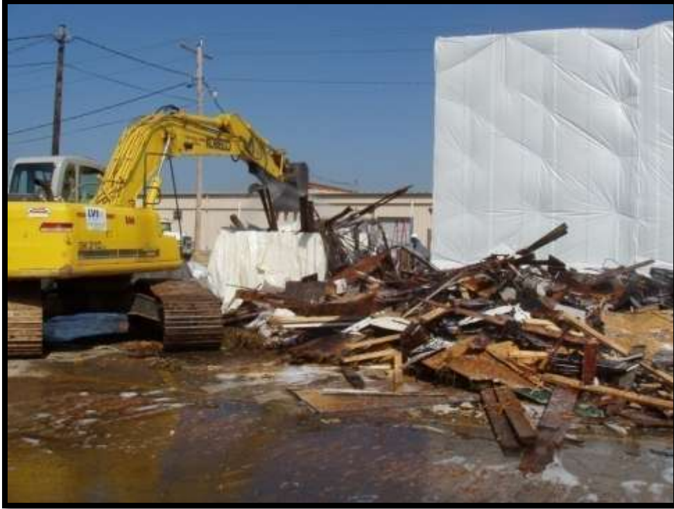
Figure 5-37. Load-out of AACM demolition debris.
