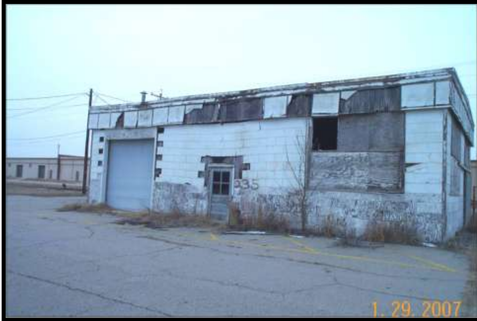
Figure 4-2. Transite building before modifications.
