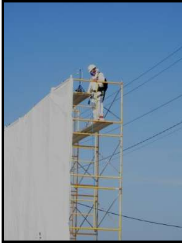
Figure 5-14. Sampling stations at the top of the barrier wall.
