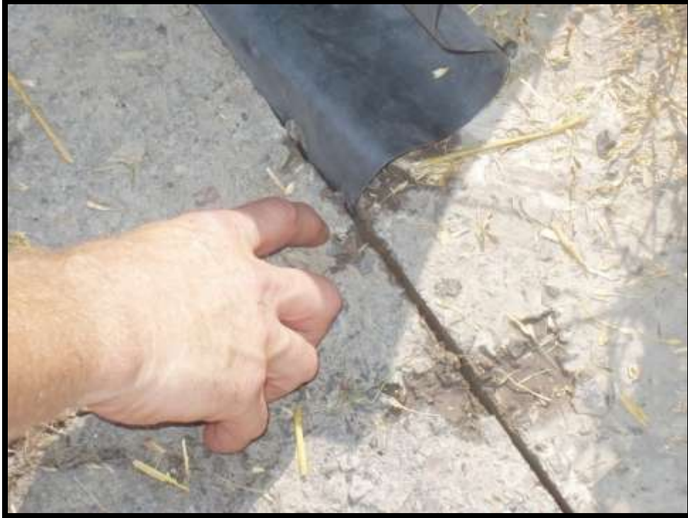
Figure 5-5. Inserting barrier into kerf in pavement.
