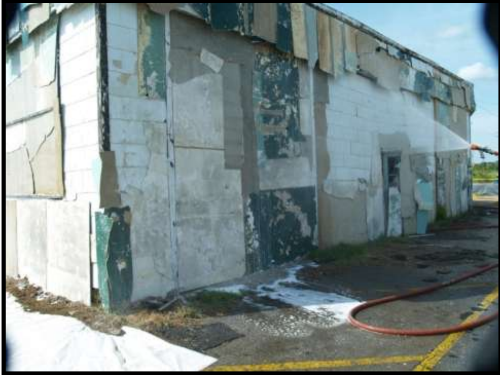
Figure 5-24. Pre-wetting of the transite building the evening before the demolition.
