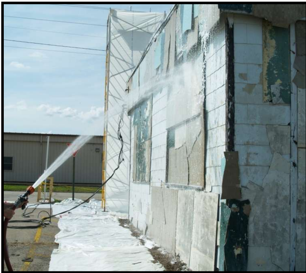
Figure 5-23. Pre-wetting of the transite building the evening before the demolition.
