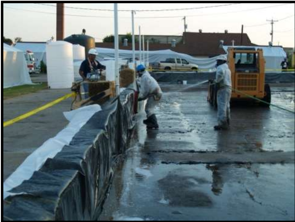
Figure 5-45. Final washing of barriers before removal.
