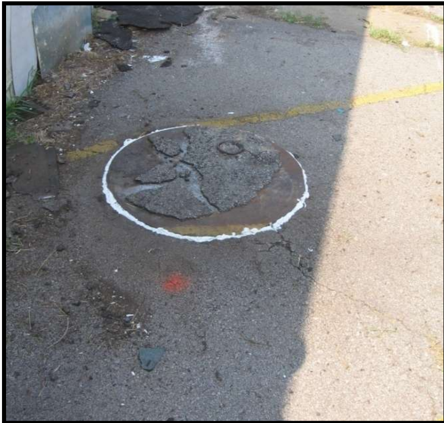
Figure 5-8. Sealed sewer access.
