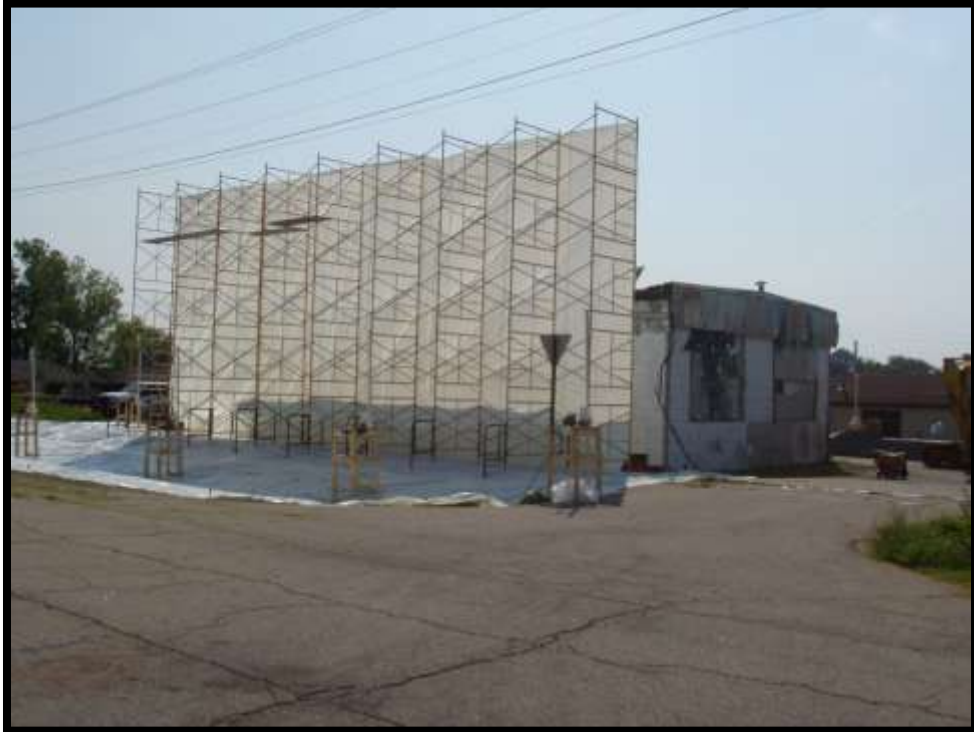
Figure 4-16. The barrier wall in place at the rear of the building.
