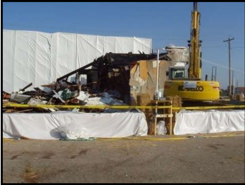
Figure 5-35. Demolition nearly complete.
