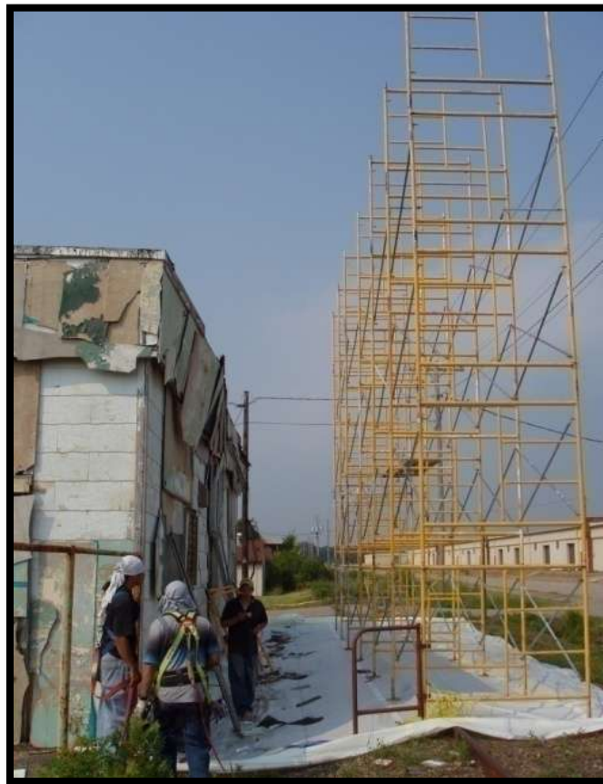
Figure 4-14. Scaffolding for the barrier wall.
