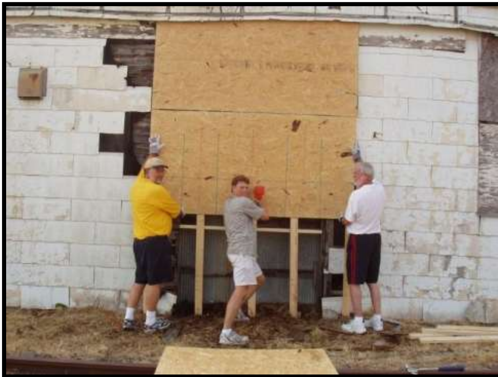
Figure 4-7. Boarding the openings to prepare for applying additional transite.
