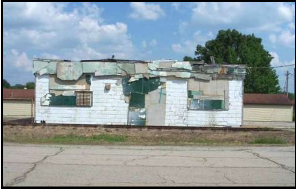
Figure 4-13. Rear view of transite building before the barrier construction.
