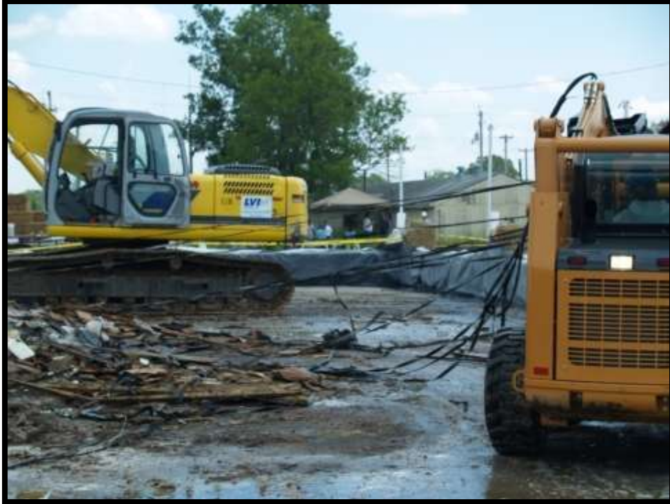
Figure 5-44. Both types of equipment were useful for debris removal.
