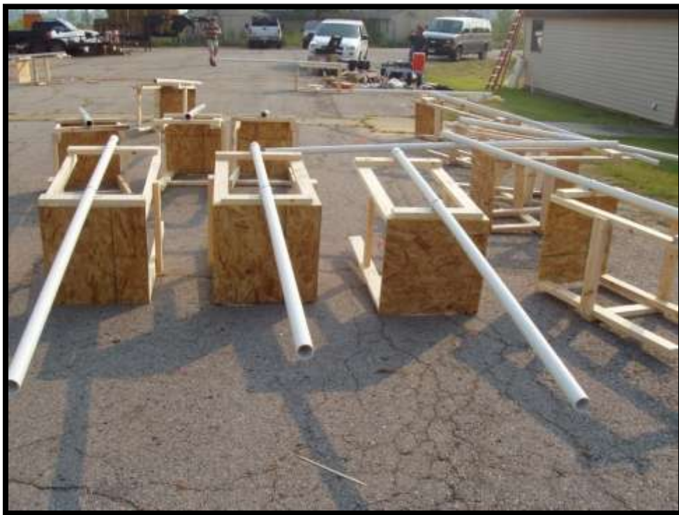
Figure 5-11. Preparation of sampling station supports.
