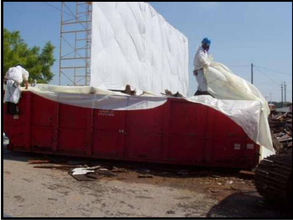
Figure 5-41. Burrito-wrapping the roll-off.
