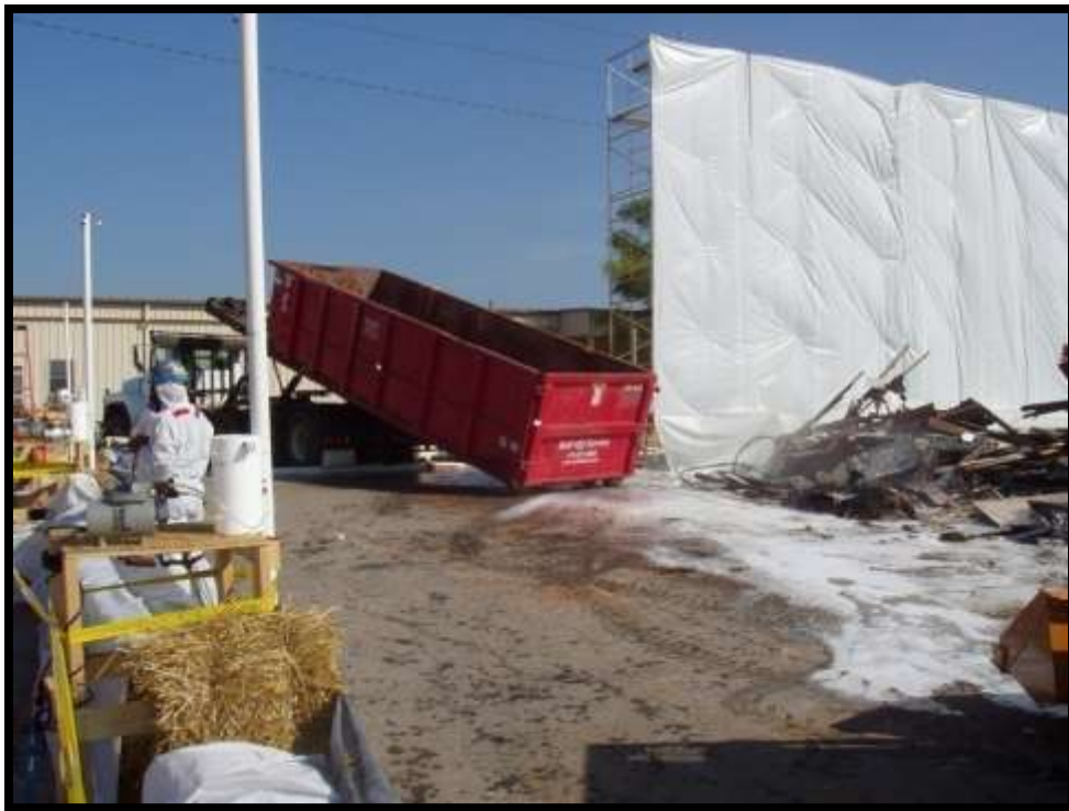
Figure 5-28. Delivery the roll-off into the site.
