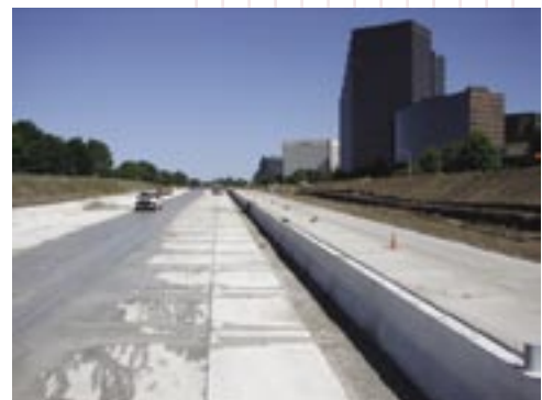
Figure 3. Lodge Freeway, Detroit, reconstructed during an extended closure for placement of jointed concrete pavement.
