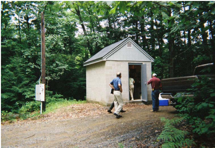
Figure 4-1. Existing Porter Well House
