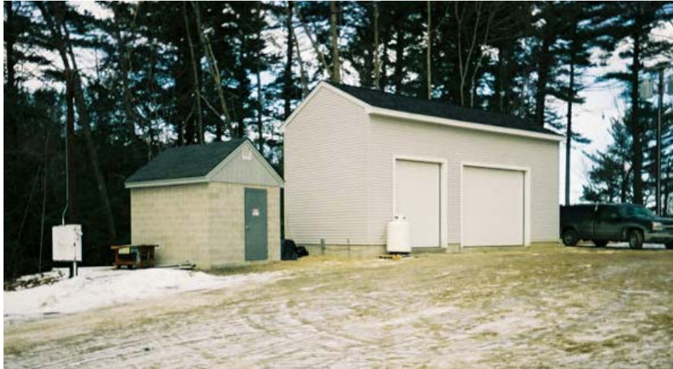
Figure 4-6. New Treatment Building (Right) and Existing Porter Well House (Left)
