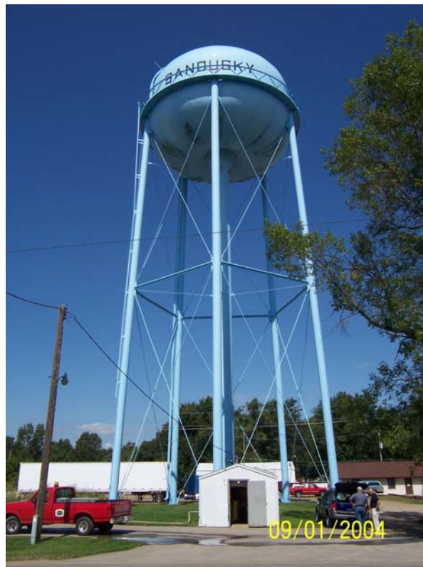
Figure 4-1. Pump House for Well No. 1 and Water Tower
