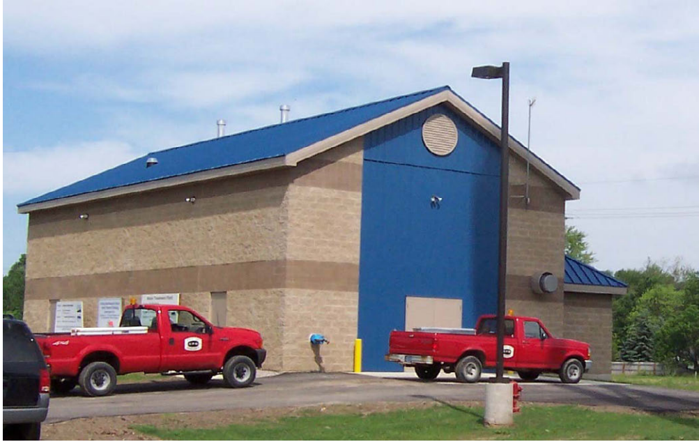
Figure 4-7. New Treatment Plant Building
