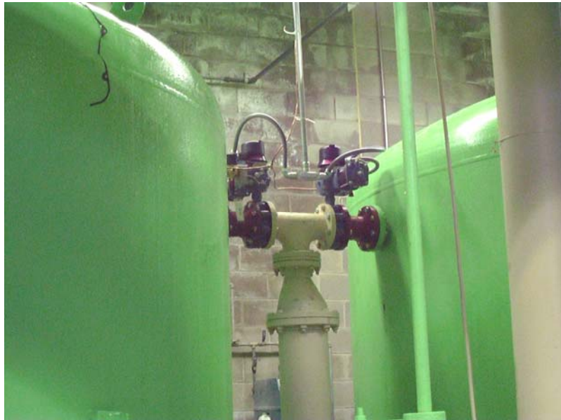
FIGURE 5-8. Pneumatically Operated Draindown Valves
