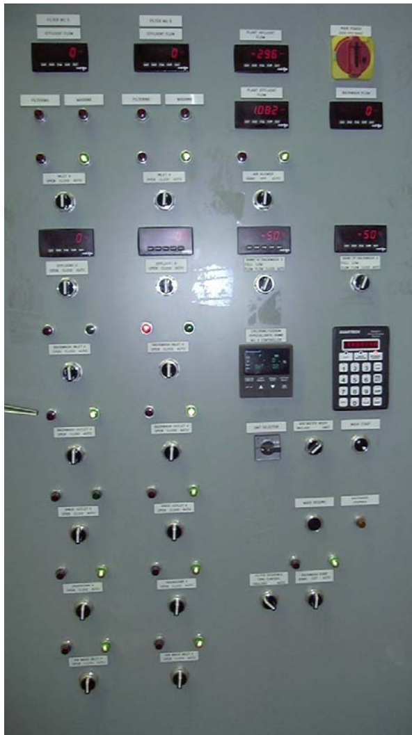
FIGURE 5-7. Typical Two-Filter Control Panel
