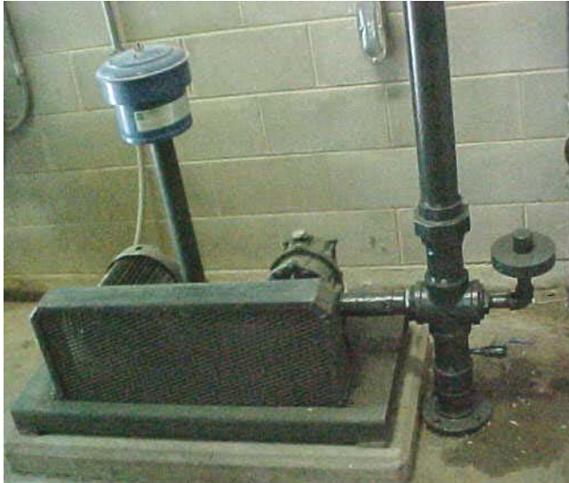
FIGURE 5-5. Air Wash Blower and Motor
