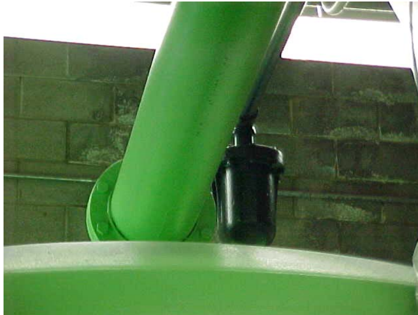
FIGURE 5-4. Air Release Valve
