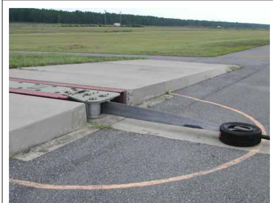
Figure A2-1. Close-up view of the Fairlead Beam and Deck Sheave.
