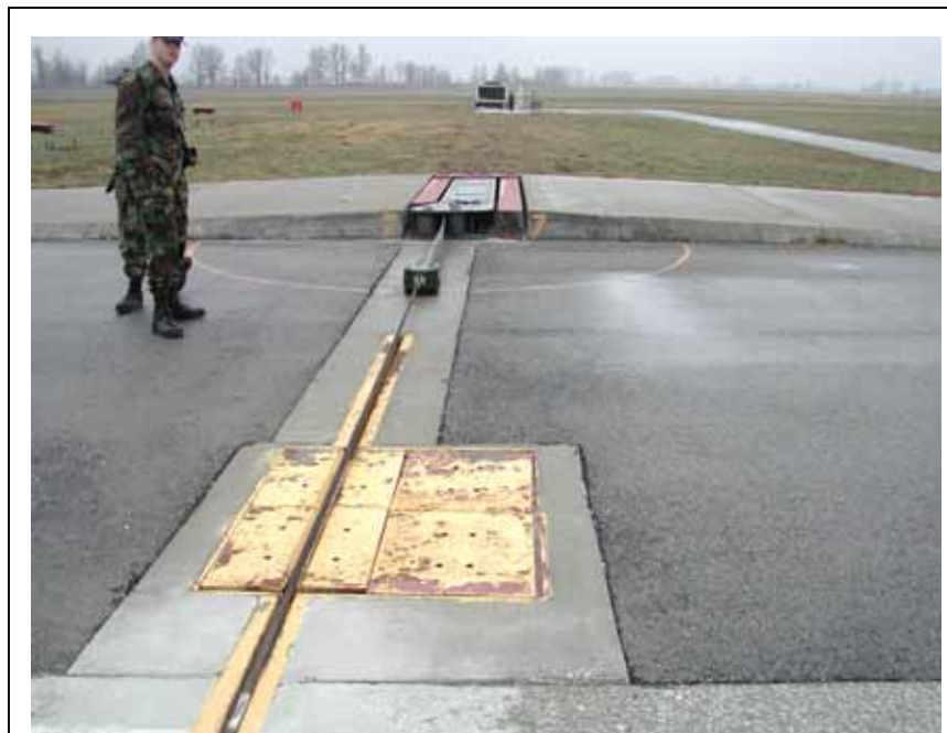
Figure A2-2. Front view of the Fairlead Beam and Deck Sheave.
