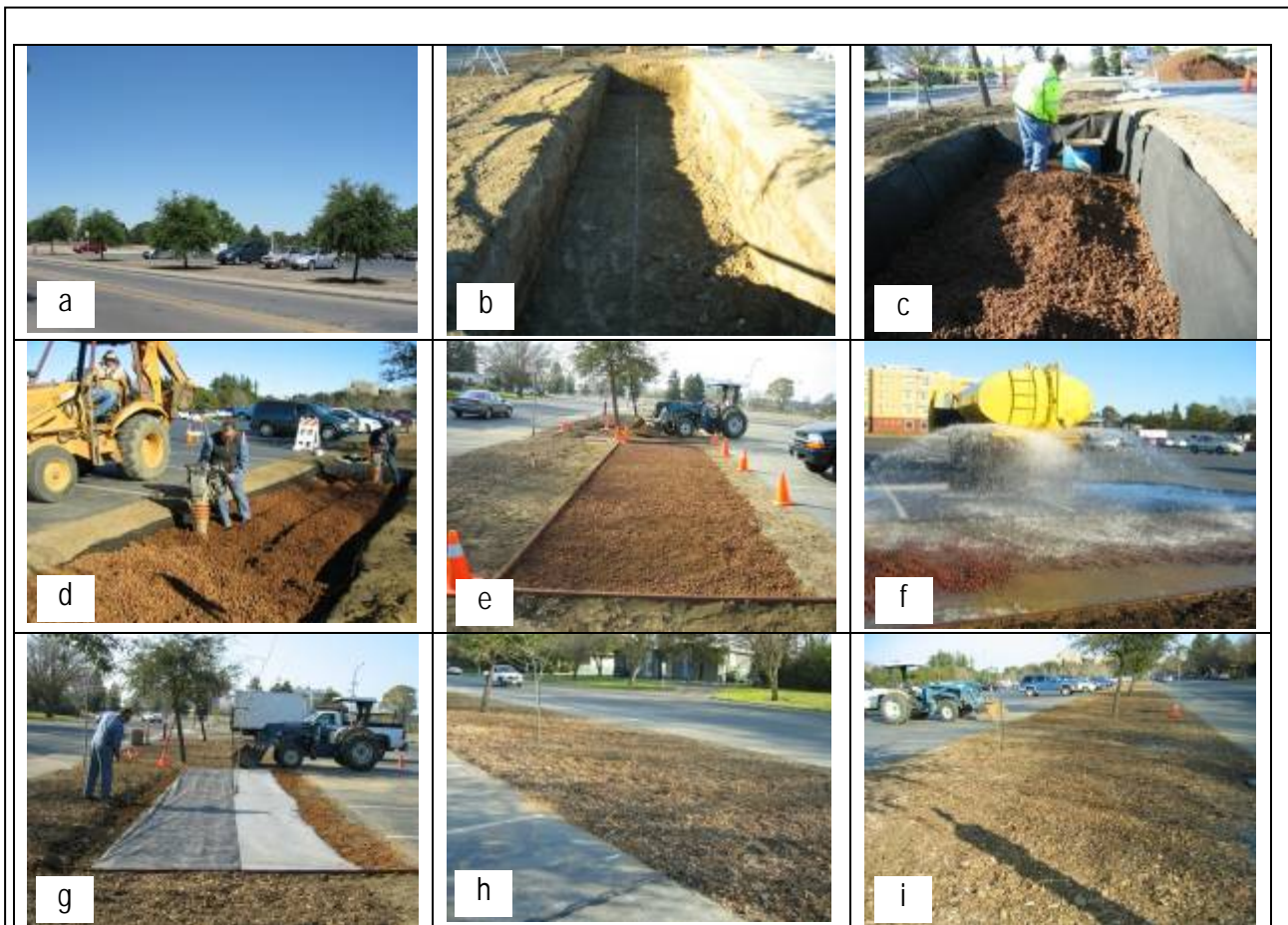
Figure 3. Field installation: a). Before GIT installation; b). Excavation; c). Fill in Davis soil; d). Compact the soil; e). Leveled the pit; f) Tested the soil settlement; g). Added tree to the system; h) Finished site; i) Both control and treatment sites were covered with mulch to match the surrounding land cover.
