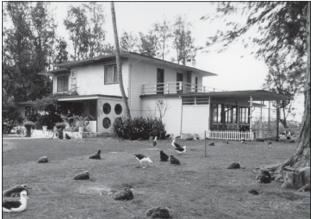
Figure 9. Officer-in-Charge house, designed by Albert Kahn (Speulda 1997).
