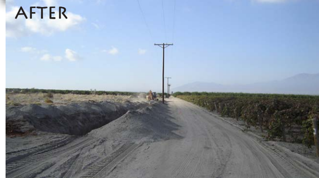
Tayawa dump site, before, during and after cleanup.
