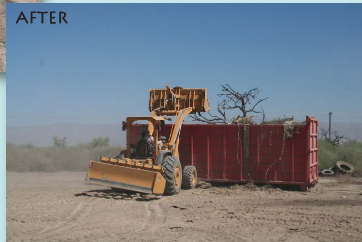
Martinez Road, before and after cleanup.
