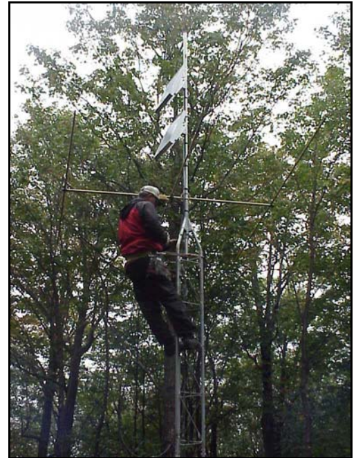
Left: Lye Brook site under construction in September 2000. Right: Don Huffman of the National Water and Climate Center works on the solar panels on the transmission antenna at Lye Brook.
