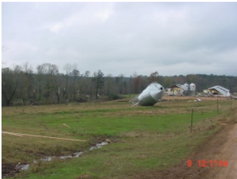
Damage to chicken farm west of Raleigh.
