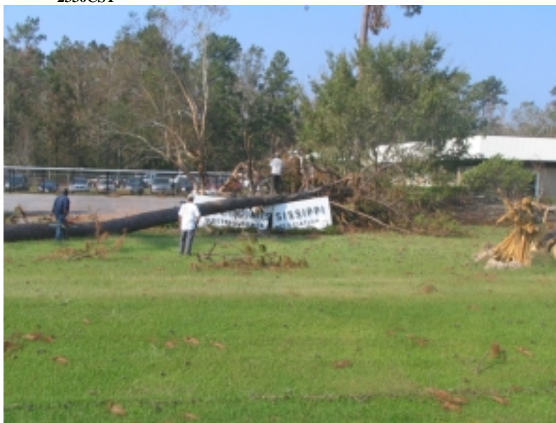
Downed trees at the South Mississippi Electric Power Association
