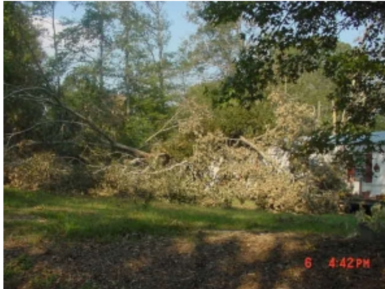
Trees downed on a mobile home just south of House.
