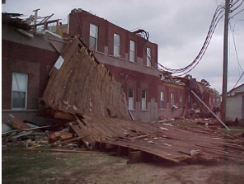
F3 damage to the Mize Attendance Center. Second floor almost totally taken off.
