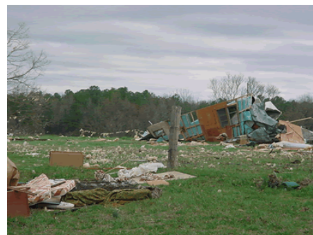
Mobile home damage on County Road 330 in Jackson County. This was caused by an F1 tornado that touched down on March 19, 2003.
