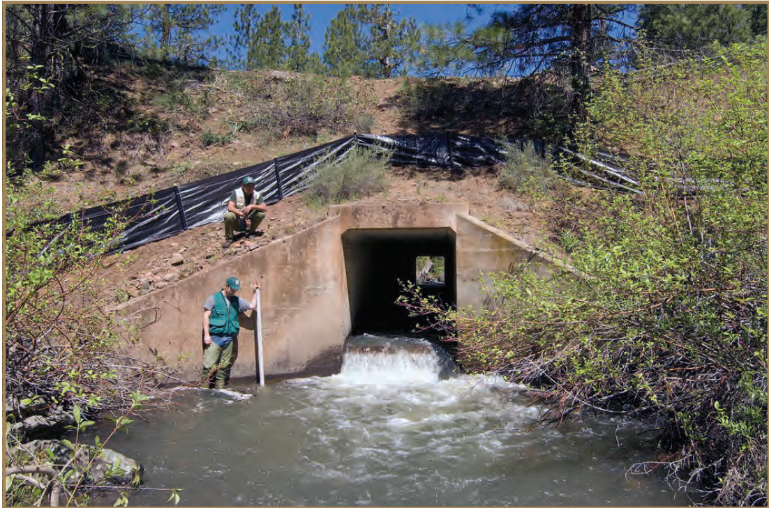
A fish passage barrier under State Highway 140 on Drew's Creek blocks access to spawning habitat for redband trout and other native fish on the Fremont-Winema National Forest, OR. Access to more than 10 miles of quality habitat was blocked by the crossing, prior to its removal.
