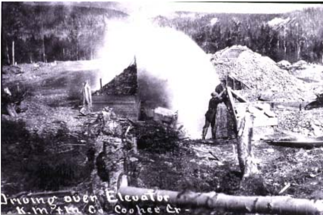
Hydraulic Mining on Cooper Creek by Kenai Milling and Mining Co., circa 1910 (Photo Courtesy Mona Painter)
