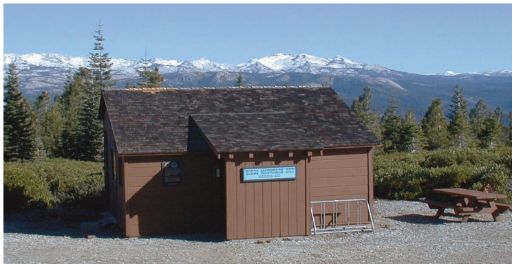
A partnership between Recreation Equipment Incorporated and the Forest Service converted the decommissioned Robbs Peak Lookout into the Robbs Hut recreation rental.
