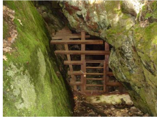
Bat gate on adit at base of Silver Mountain
