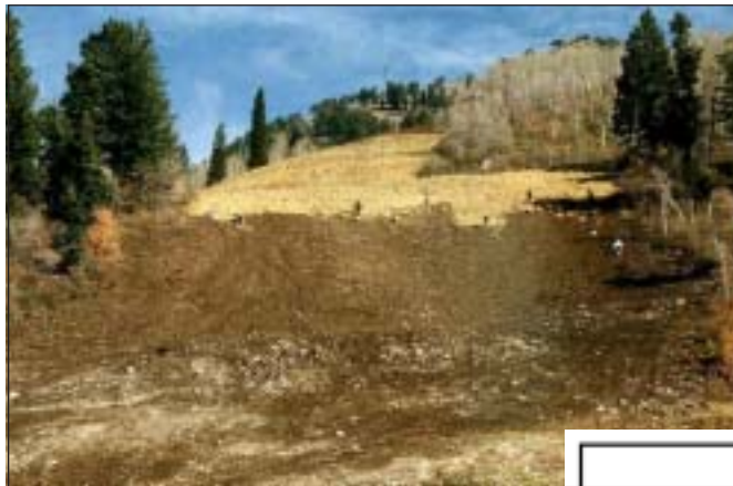
Straw mulch application by hand crews on larger ski slopes is a time consuming task.
