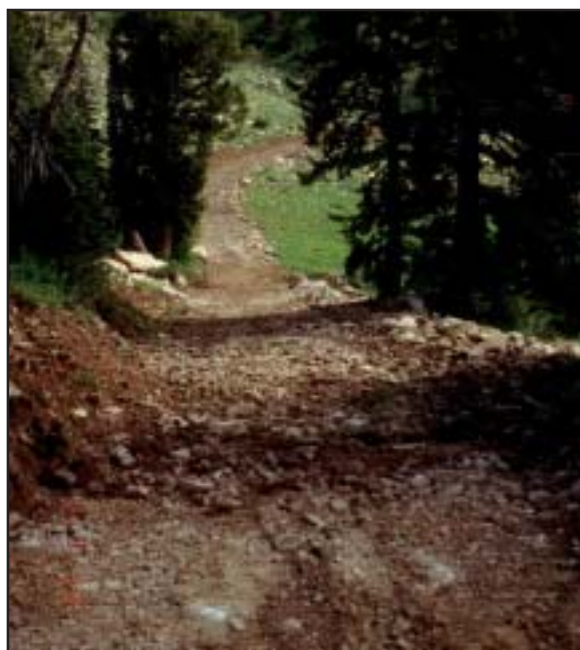
Water bars used to divert water off road surfaces must be shallow and wide to allow vehicle passage.
