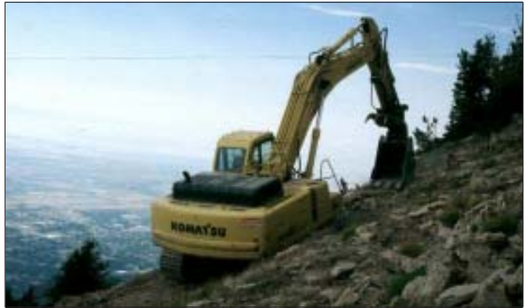
Full bench cut and end haul construction of a narrow low standard access trail.
