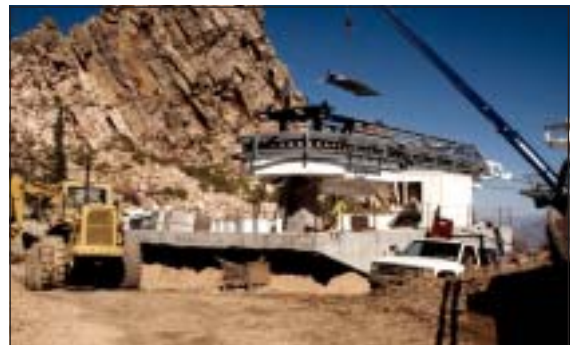
Excavations for ski lift terminal building foundations can yield large amounts of material that can be salvaged as fill for other activities.
