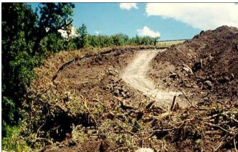
Where space is limited, less effective practices such as berms, silt fences, and slash barriers can be used together to replace a vegetation buffer strip.
