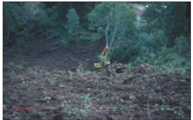
Vegetation clearing by trackhoe excavator leaving root mass and coarse debris ground cover.
