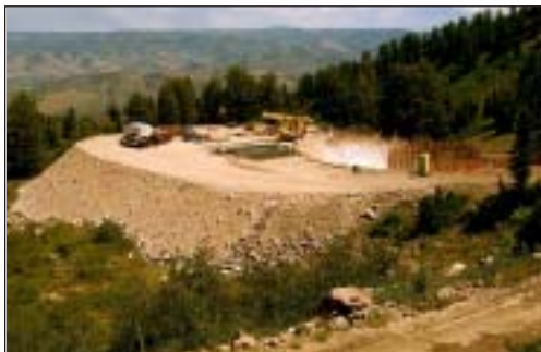
Storage tanks can generate large amounts of excess excavated material that must be wasted in some location or hauled off of the mountain.
