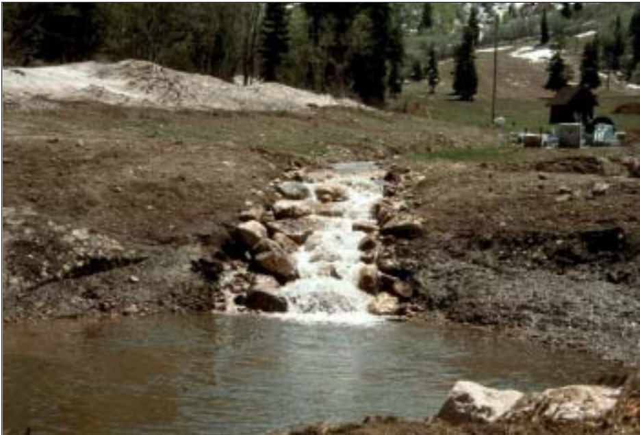
Detention basin inlet channels should be protected from high flows and head cutting with rock riprap and flow control gates.
