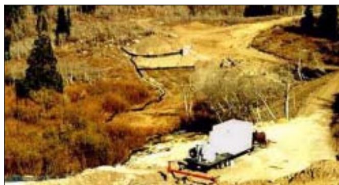
Wetlands should be protected from sediment sources with buffer strips of live upland vegetation.
