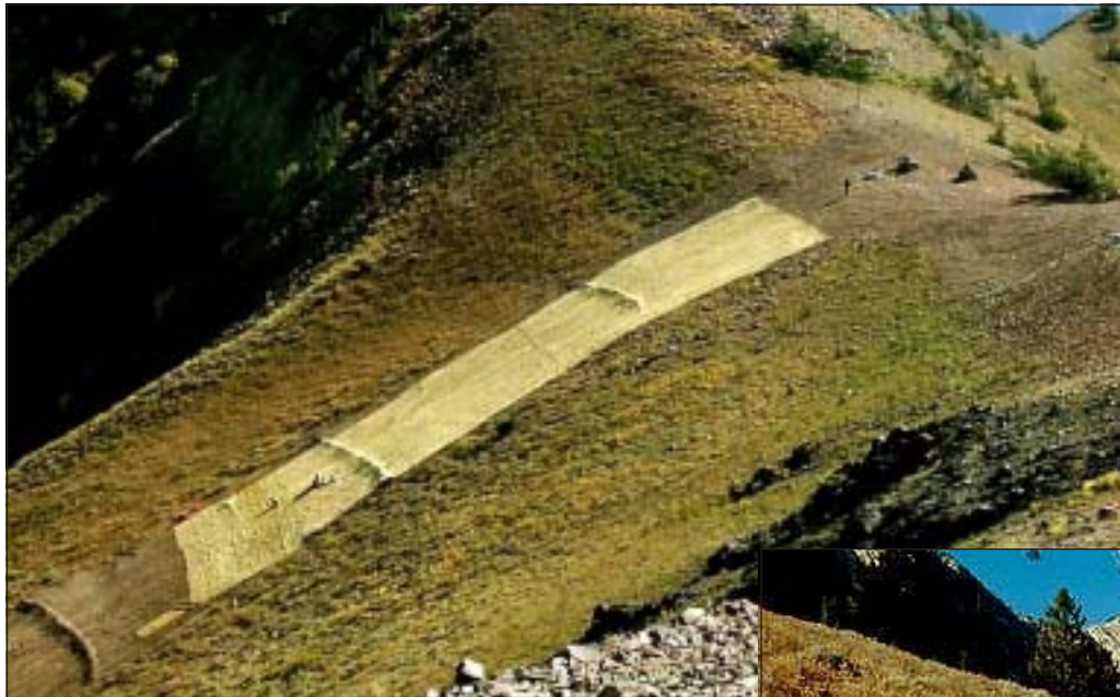
Although more expensive to purchase than straw, mulch blankets install much faster and are more durable.
