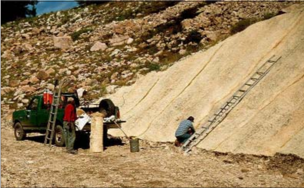
Successful revegetation on harsh sites, such as over-steep and erosive slopes, requires a durable mulch blanket cover.
