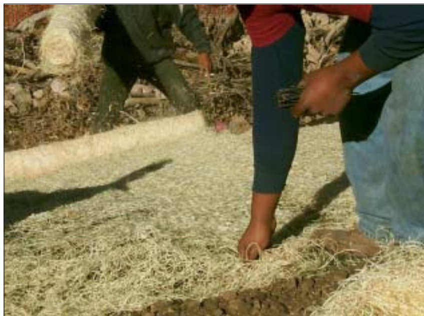
Blankets must be properly stapled in place to resist lifting and tearing by strong winds.
