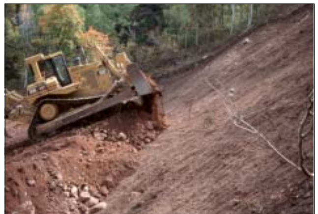
Swales and slope break compressions can be smoothed out by filling with subsoil excavated from building and lift terminal foundations.
