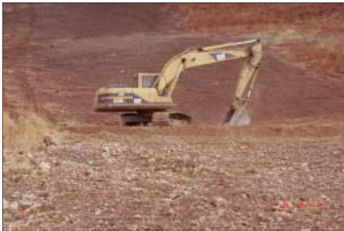
Waterbar installation by trackhoe excavator.
