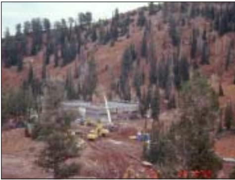
Mountain buildings can be tucked into hillsides and away from streams, allowing for vegetation strips to filter sediment and runoff.
