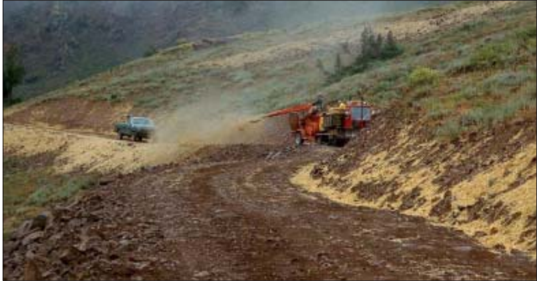
Road cut and fill slopes can be quickly covered with mechanical mulching equipment.
