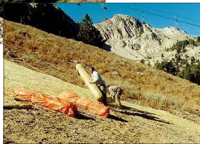
Mulch blankets are commonly made from wood or straw fibers and stitched to an open weave net. Either type of blanket is very light and easy to handle and transport across rough terrain.
