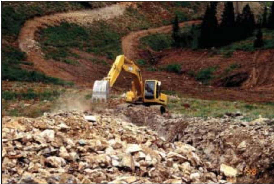
Topsoil is a scarce resource in many mountain environments. Trench excavation should salvage topsoil where present to use in restoration work.
