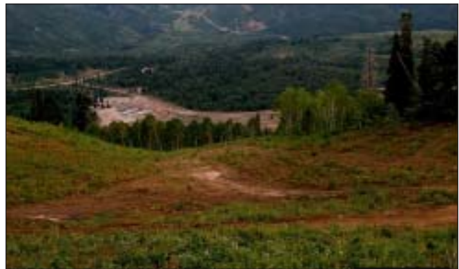
Disturbances from multiple entrances into newly reclaimed areas should be kept as small and narrow as possible.
