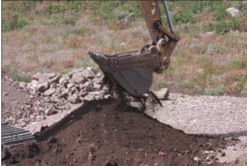
Screened trackhoe buckets work well to separate out and salvage valuable topsoils.
