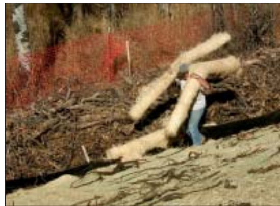
Blankets can be combined with silt fencing to provide added protection next to streams and wetlands.
