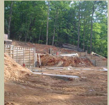
Mountain Home Construction
