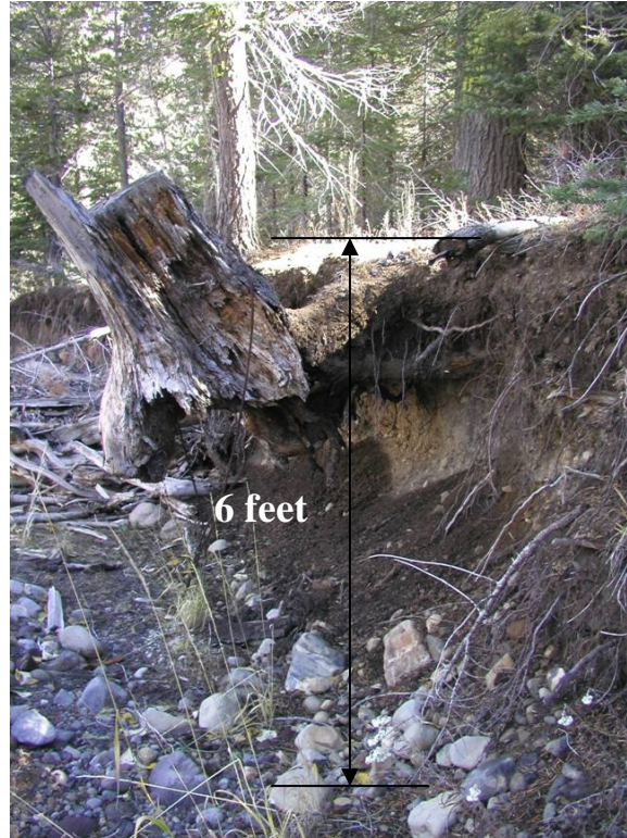
Unstable, vertical cut-bank located just downstream of the head cut knick point near the upstream end of Site B
