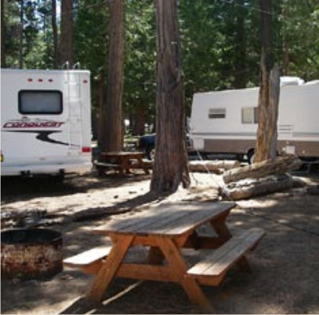
Many campground sites have old utility hookups and need upgrades for accessibility.
