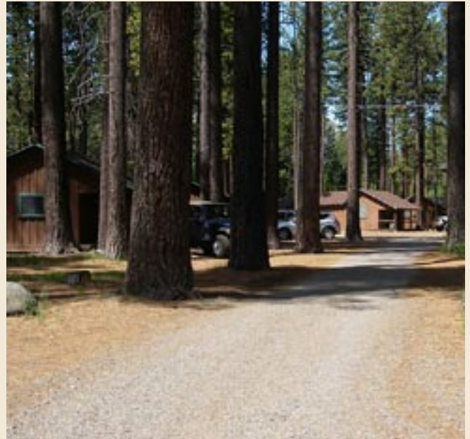
Existing cabin facilities need to be restored and some replaced to provide code compliant facilities for the public.
