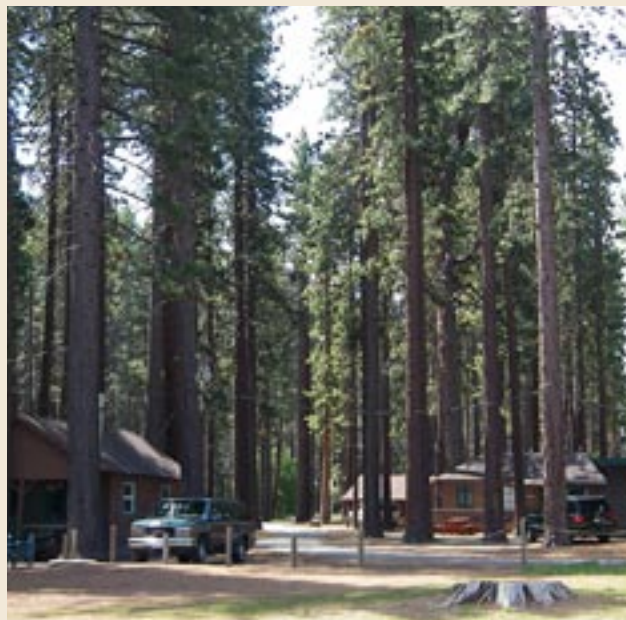
A range of cabins have been constructed. Some have historic significance and many require replacement.
