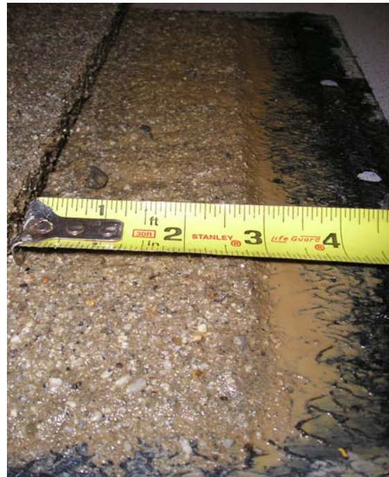
Completed test showing sand and geomembrane. Drained, FML sample taken out of box, no top box.
