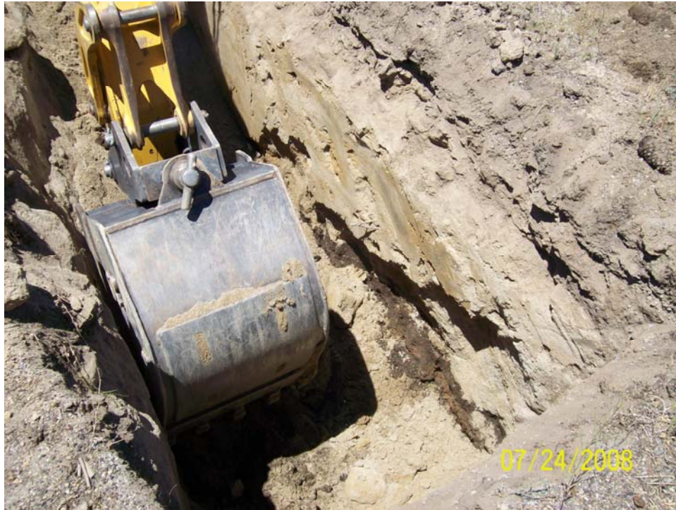
Photograph A-3. USFS – Meyers Landfill – Excavating ML-TP-02 PERC-1. Photographed: July 24, 2008
