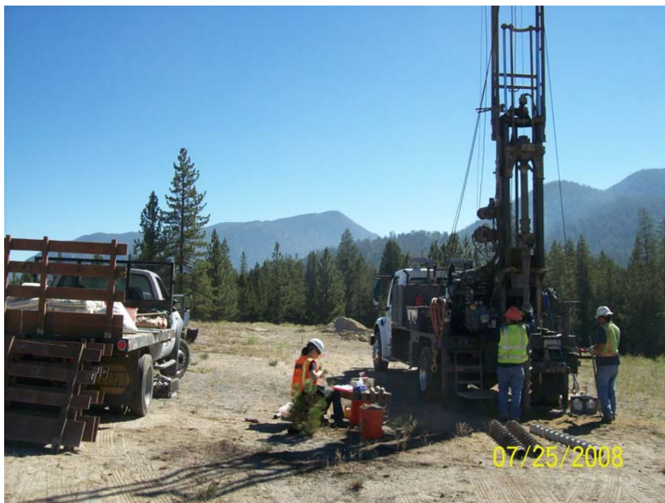
Photograph A-14. USFS – Meyers Landfill – Drilling geotechnical boring ML-SB-01.
