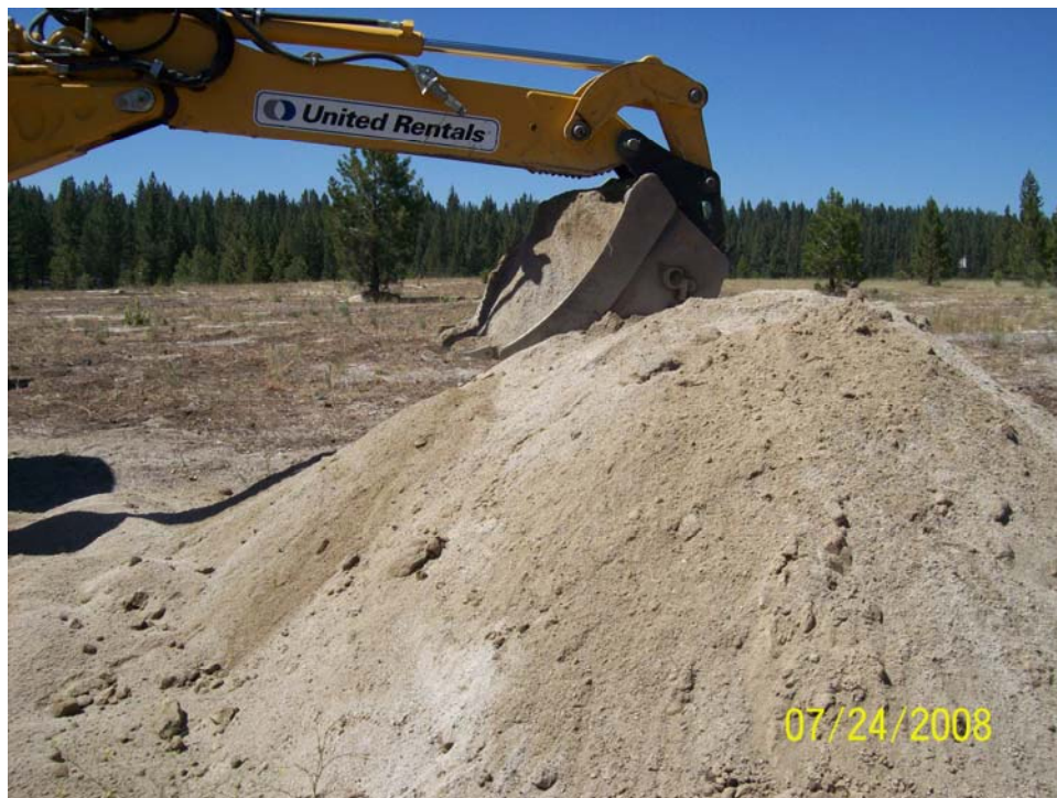
Photograph A-5. USFS – Meyers Landfill – Stockpiled spoils from ML-TP-01. Photographed: July 24, 2008
