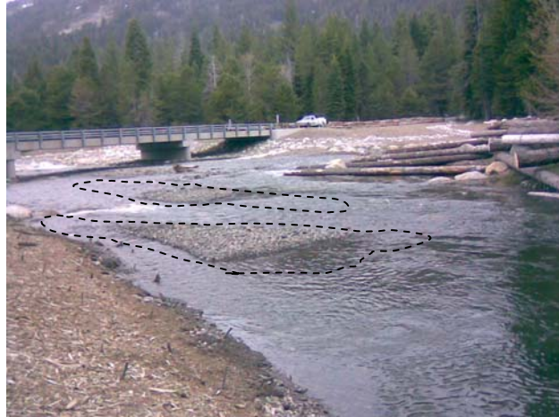
Figure 5. Lateral bar formation downstream of bridge
