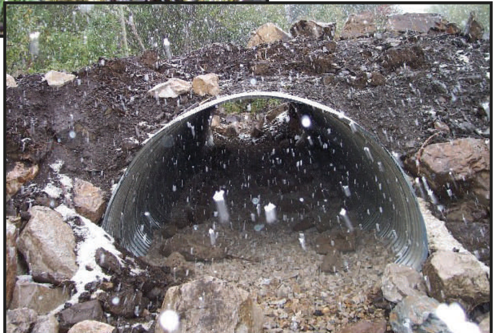
Upper Gance Creek crossing. Post-implementation. Looking upstream at culvert (squash: 83" by 57").
