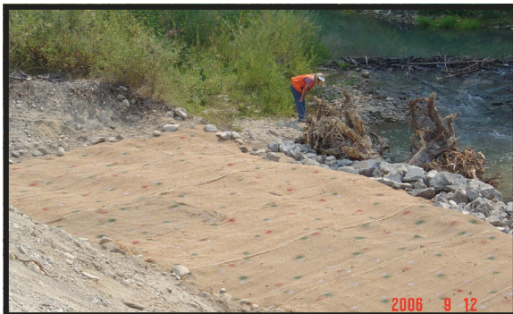
Large, woody debris fish structure with bank rehabilitation.
