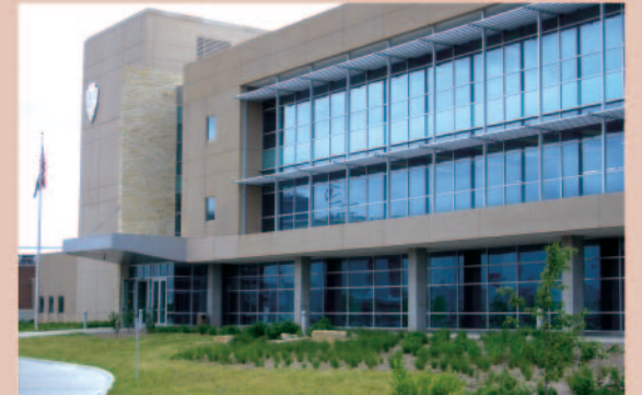
LEED-NC Gold National Park Service Midwest Regional Headquarters, Omaha, Nebraska
