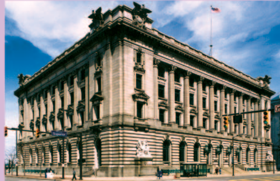
Metzenbaum U.S. Courthouse, Cleveland, Ohio
