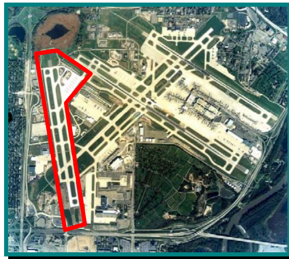
New runway 17/35 Complex at Minneapolis-St. Paul International Airport.
