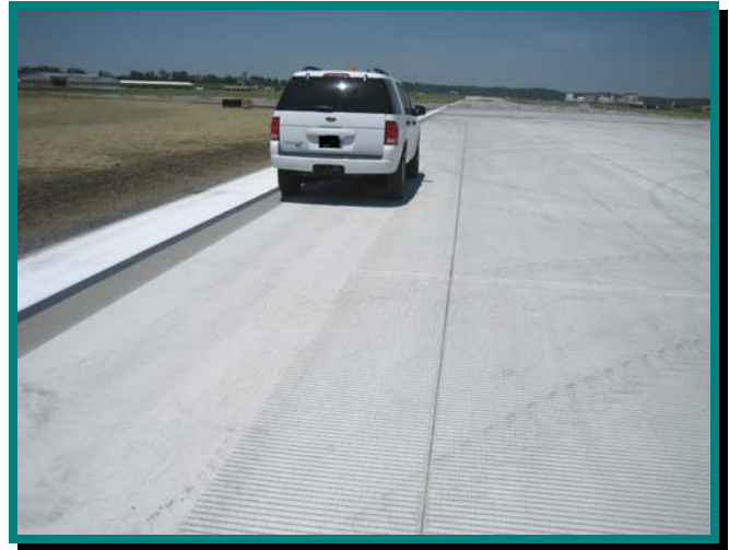
Pavement in good condition.
