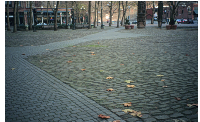
Figure 4-35. In Pioneer Square in Seattle, Washington, an additional pathway was created using smoother and larger pavers with fewer changes in level.
