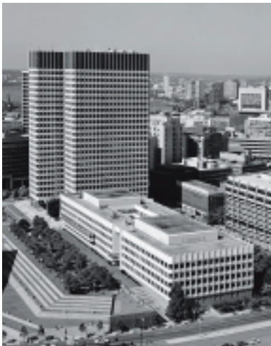
JOHN F. KENNEDY FEDERAL BUILDING, BOSTON, MASSACHUSETTS | WALTER GROPIUS AND THE ARCHITECTS COLLABORATIVE | 1964-66
