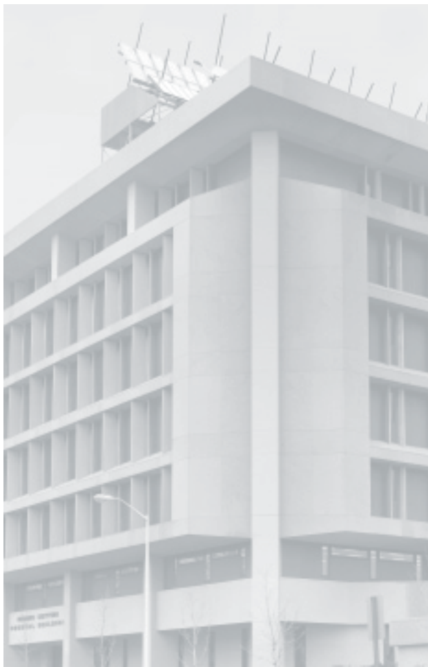
NORRIS COTTON FEDERAL BUILDING, MANCHESTER, NEW HAMPSHIRE | ISAAK & ISAAK | 1976
