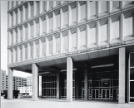
ENTRANCE SHOWN BEFORE UPGRADES (ABOVE), AND AFTER UPGRADES HAD BEEN COMPLETED (UPPER RIGHT).
