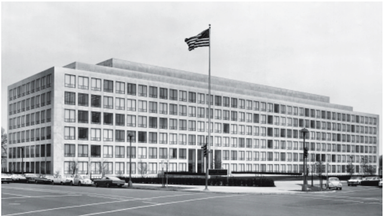
FEDERAL OFFICE BUILDING 10B, U.S. DEPARTMENT OF TRANSPORTATION, FEDERAL AVIATION ADMINISTRATION, WASHINGTON, DC | HOLABIRD, ROOT & BURGEE AND CARROLL, GRISDALE & VAN ALLEN | 1963
