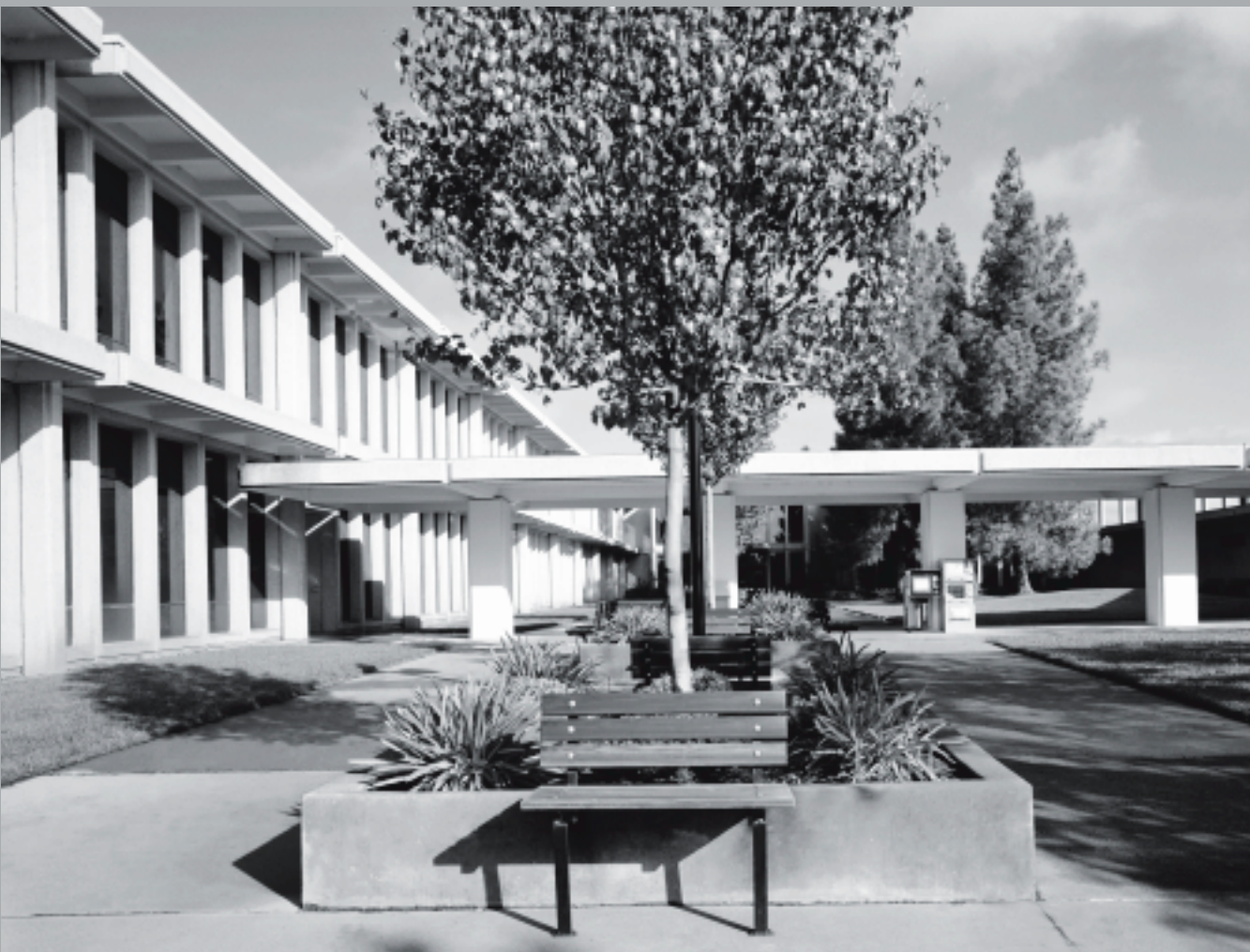
FEDERAL BUILDING, SACRAMENTO, CALIFORNIA | DREYFUS & BLACKFORD | 1967
