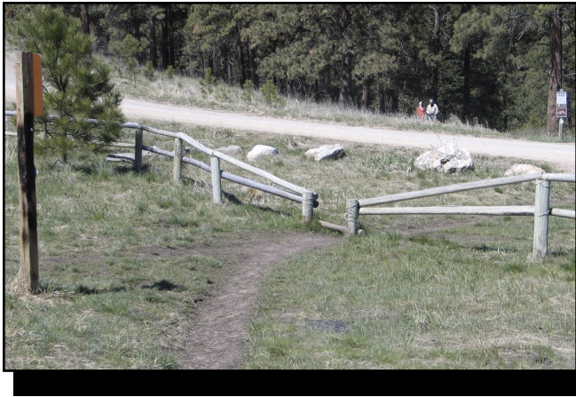
Figure 6—A gate in the Lolo National Forest that allows horses to pass, but restricts ATVs. This gate is not accessible because it is narrower than the minimum width required for passage of a wheelchair (32 inches) and the bar across the opening is higher than 1 inch.
