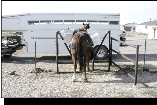
Figure 4—A horse walking through a “V” gate in Utah. This gate is not accessible because it is narrower than the minimum width required for passage of a wheelchair (32 inches) and the bar across the opening is higher than 1 inch.
