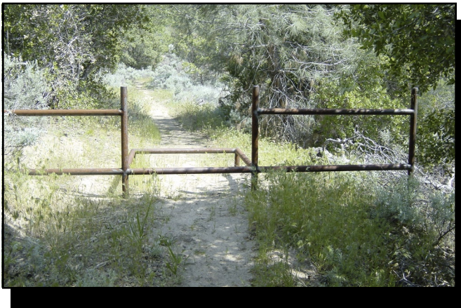
Figure 7—A horse stile. This gate is not accessible because the bars across the opening are higher than 1 inch.
