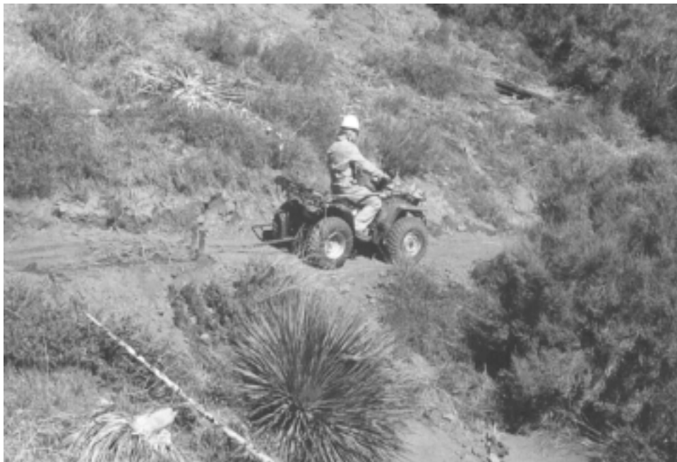
Figure 31A.—ATV dragging a harrow, Pacific Crest Trail, Angeles National Forest.
