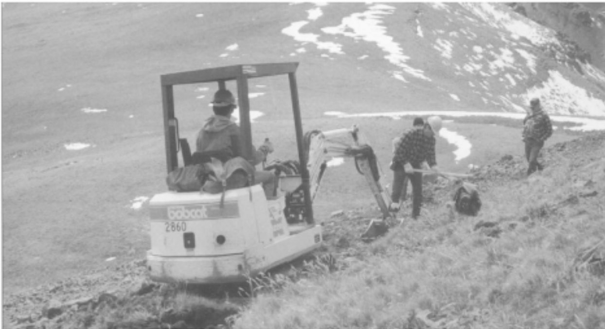
Figure 2.—Bobcat compact excavators construct trails throughout the Rio Grande National Forest.
