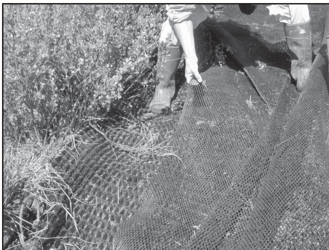
Figure 14—Polynet over Pyramat was used in this National Park Service installation to test the addition of a synthetic turf reinforcement mat. The Polynet, with its more durable wear surface, was installed over the less durable Pyramat.
