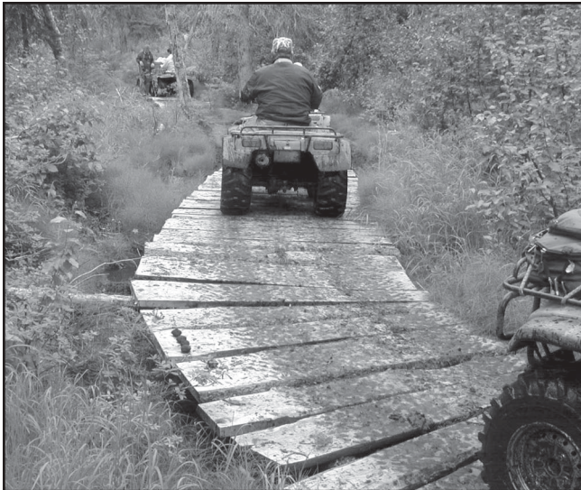
Figure 20—A finished puncheon trail. Note the placement of the plank taper to accommodate the curves along the trail.
