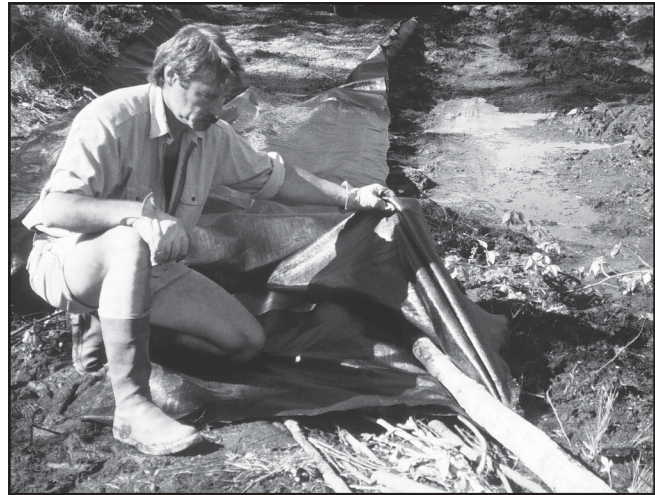
Figure 11—The author installing woven geotextile around a rim log in the geotextile gravel-capping test installation at the Yukon-Charley Rivers National Preserve in Alaska. The rim log held the gravel cap on the installation.
