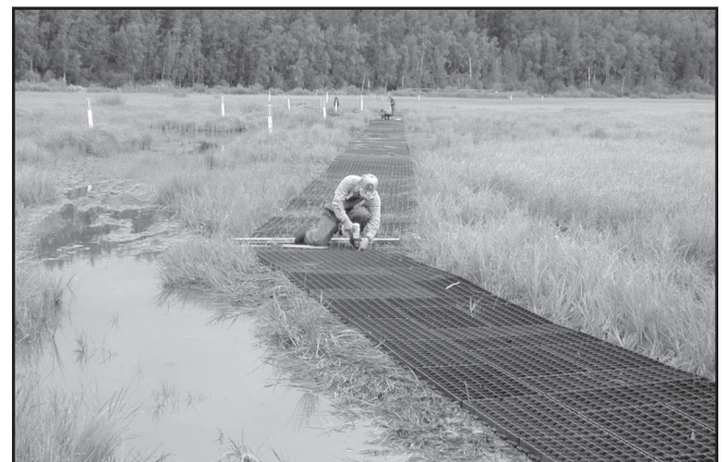
Figure B8—Angular cuts in the panel sections help form the turns in the trail.
