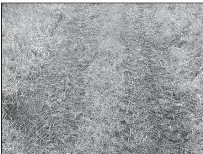
Figure 15—A Park Service Polynet/Pyramat test installation after 3 years in a wetland area with a high percentage of sedge. By the third year, sedge had become well established and its roots well entwined with the Pyramat matting.
