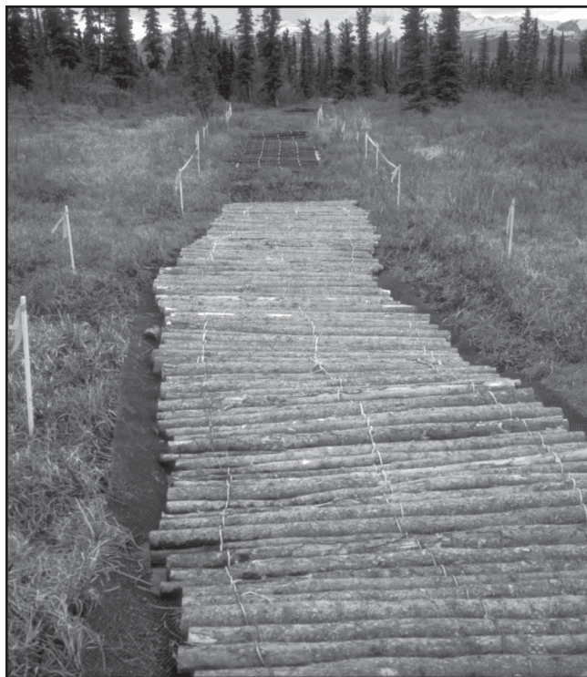
Figure 16—Spruce pole corduroy laid across permafrost soils in Alaska. These poles were imported to the site and secured by weaving them with three strands of \frac{3}{8} -inch nylon line.
