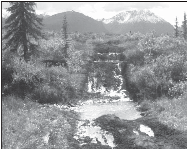
Figure 1—A degraded trail in interior Alaska. Heavy use has stripped surface vegetation and exposed permafrost soils to accelerated melting, resulting in muddy, rutted trail surfaces, erosion, and deep muck holes.
