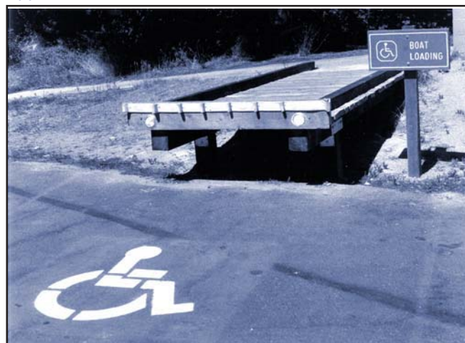
Figure 10—Reflectors are recommended for loading platforms.
