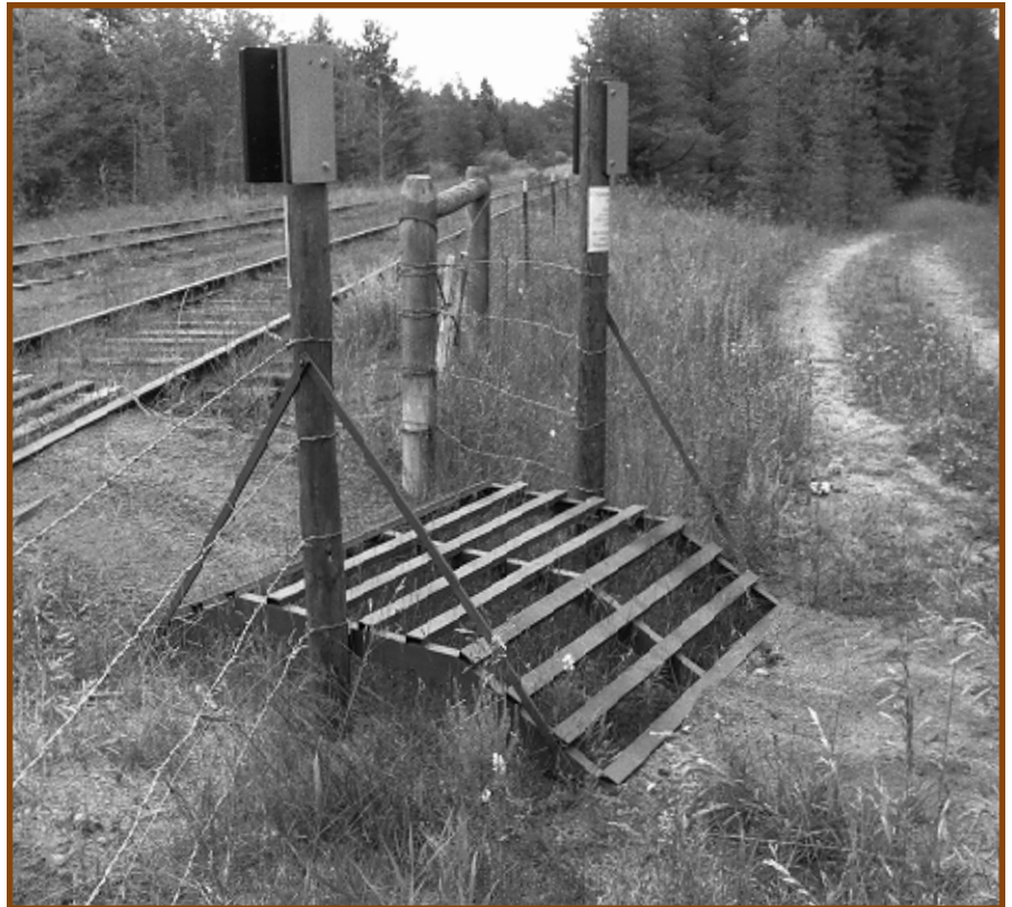
Figure 3—The side supports (or wings), extending from the Deerlodge Trail Cattle Guard to the fencepost, are essential in persuading cattle not to jump the cattle guard. Butting the posts up to the cattle guard helps keep vehicle speed down, but at the risk of catching handlebars.
