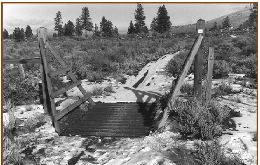
Figure 2—For safety, you will absolutely want a straight approach on either side of the cattle guard. Modify the fence or the trail, if necessary, to ensure the approach is straight. Curves in the trail leading to the approach can help reduce speed. Note the gate to the right of the cattle guard for horse riders and livestock.
