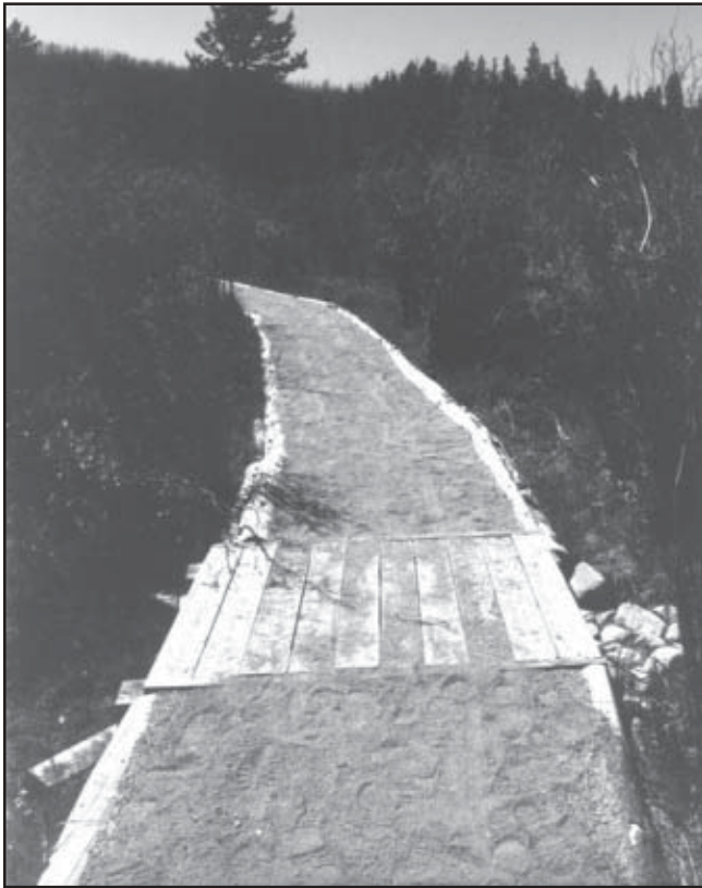
Figure 17—A new turnpike will need additional fill as it settles, especially during the first year. This turnpike has a timber culvert.
