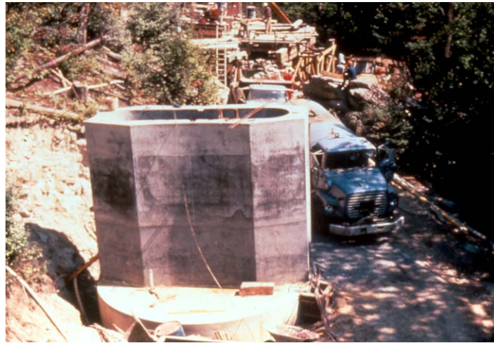
Figure 1.19 – Precast Hollow Segmental Piers, Linn Cove Viaduct, North Carolina
