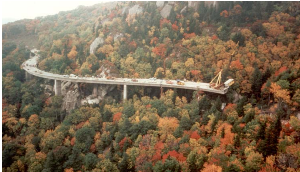
Figure C.9 – Construction of the Linn Cove Viaduct
