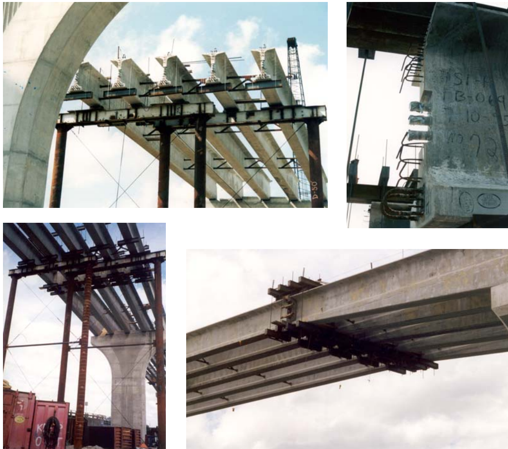
Figure 1.7 – Spliced Haunched I-Girder of Main Span Unit.
