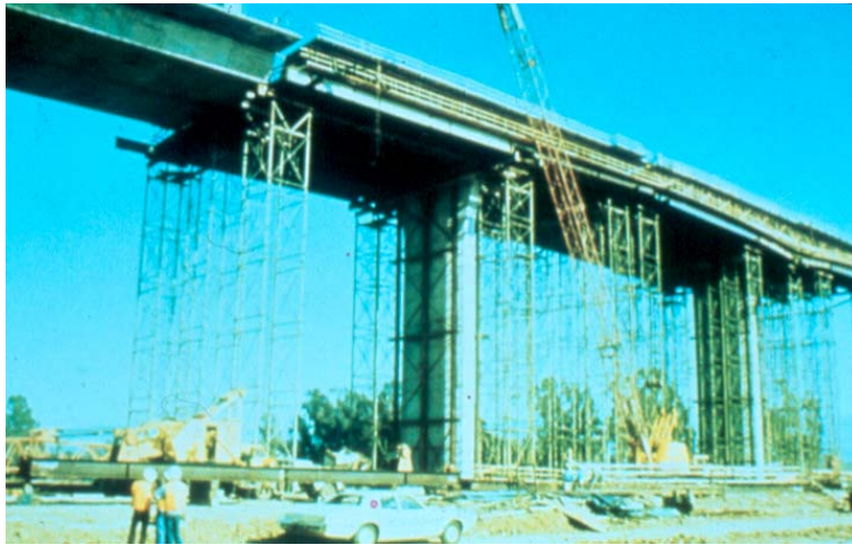
Figure 1.6 – Cast-In-Place Post-Tensioned Construction in California.
