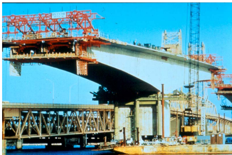
Figure 1.9 – Cast-In-Place Segmental Construction using Form Travelers
