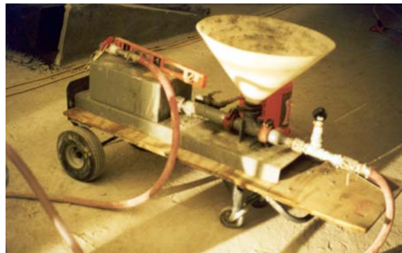
Vacuum Grout Injection
