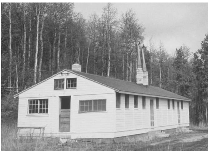
The Pole Creek Ranger Station Bunkhouse (pictured here in 1959) on the Humboldt-Toiyabe National Forest originally served as a CCC barracks at Camp Antelope in Coleville, California.
