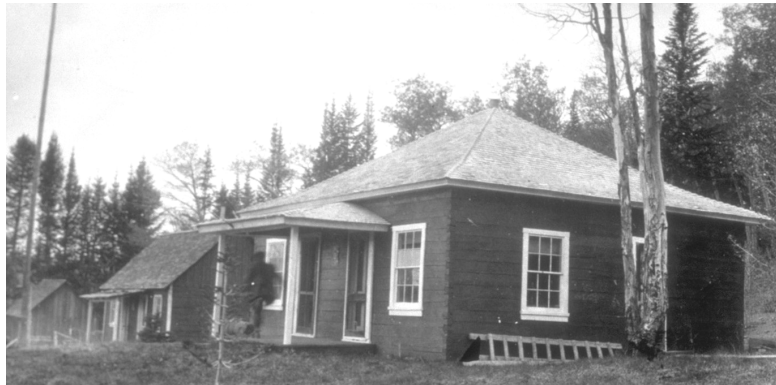
Koosharem Ranger Station, Fishlake National Forest, was constructed of the 1908 standard plan #12.
