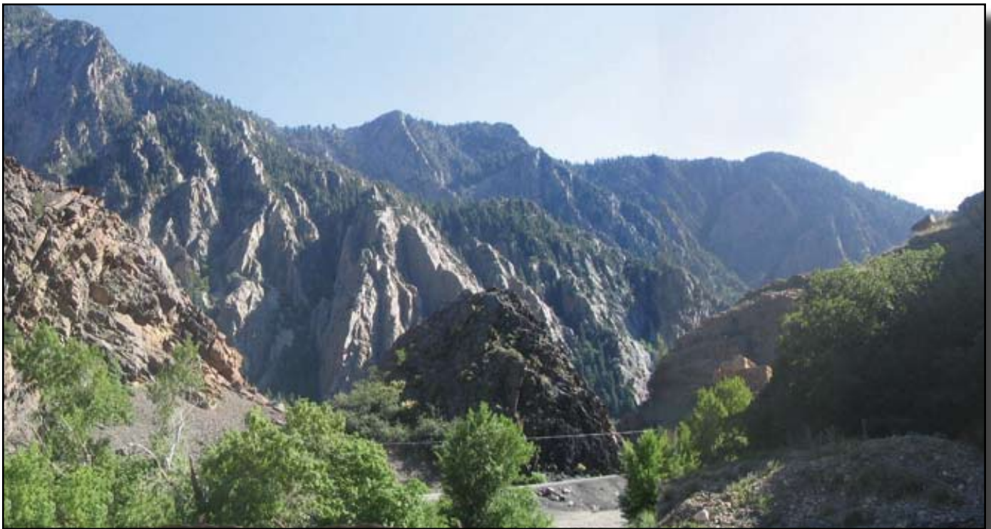
Located just east of the Storm Mountain slide area, this site is at the water diversion facility for the Big Cottonwood Canyon hydropower plant. View looking south. D. Prevedel photo July 8, 2005
