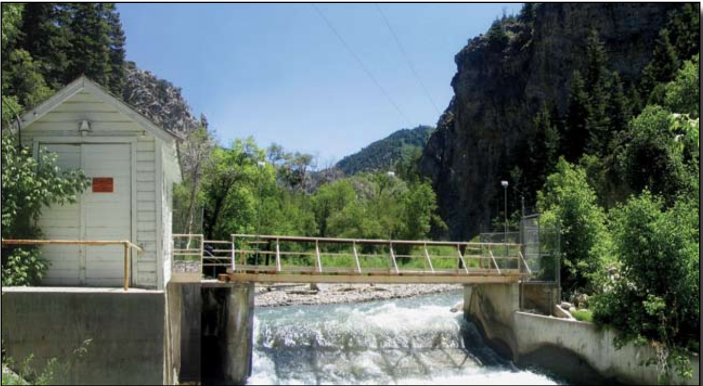
This site is now at the UPL diversion, one quarter mile west of Little Mill Campground. View looking east. D. Prevedel photo July 8, 2005
