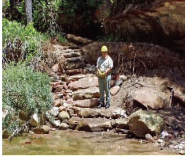
Construction of rock stairs at West Fork trail
