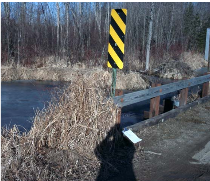
Moss on deck ends, damage to upstream stringer and railposts
