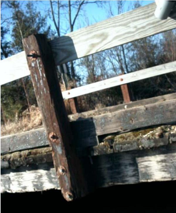
Moss on deck ends, damage to upstream stringer and railposts
