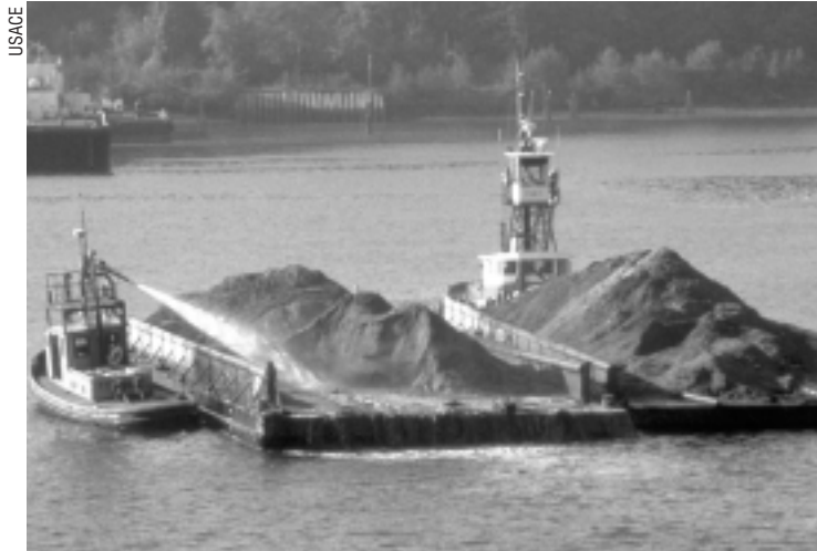
As ships increase in size and the need to deepen ports and waterways grows, economical and environmentally friendly ways to dispose of dredged material pose a major challenge.
