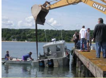
Ashland FRO's Research Vessel CHUB developed a cracked hull in rough seas during a whitefish assessment survey in Lake Superior. With help from some local agencies and businesses, the CHUB was lifted out of the water and repaired.
