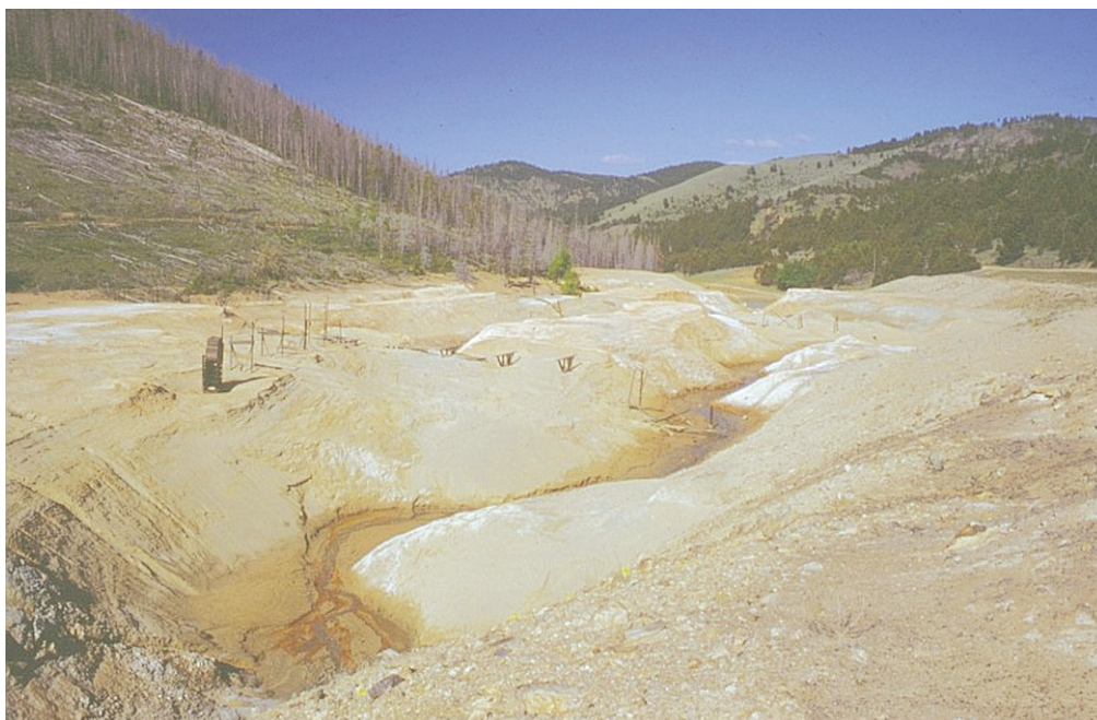
Figure 2. Mill tailings in High Ore Creek valley at Comet mine site before large-scale remediation activities, October 1996. Photograph by D.A. Nimick.
