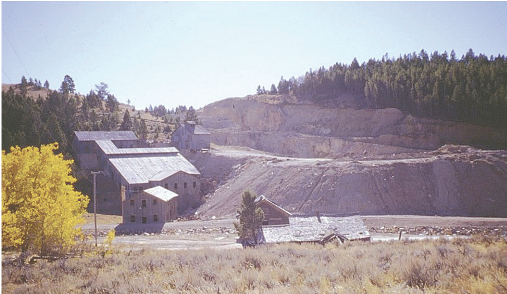
Figure 3. Comet Mill and open-pit mine before large-scale remediation activities, October 1996. Photograph by D.A. Nimick.
