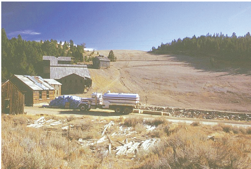
Figure 5. Comet Mill and mine site after remediation activities, August 1998. Waste rock and tailings have been removed, and the open pit has been used as a repository. Photograph by D.A. Nimick.
