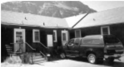
Entry to public showers, General Store/Motel at Rising Sun
