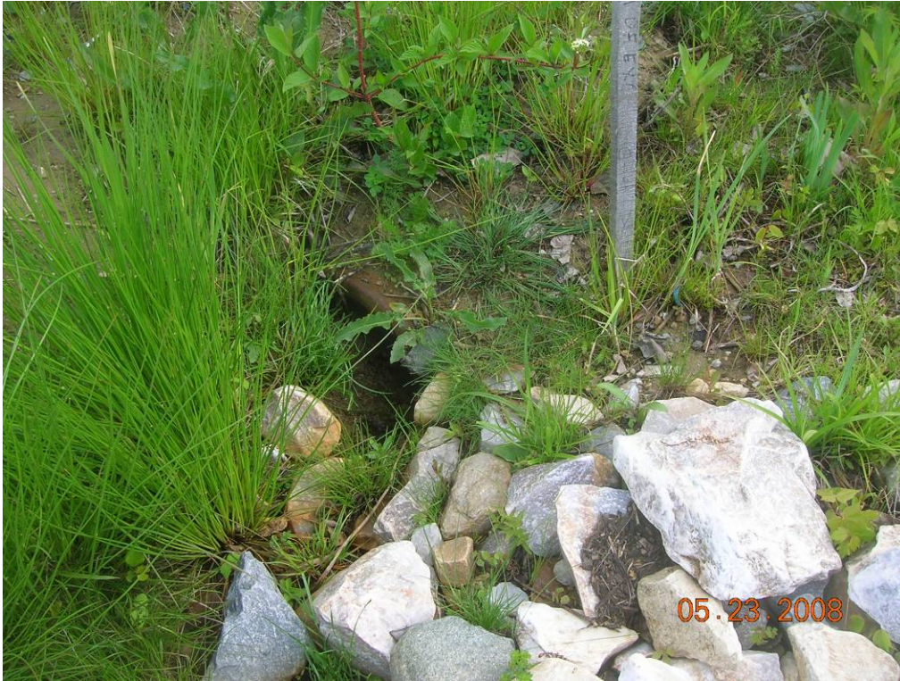
Photo 6 - GE Location 4 - View of the location of the 20-inch outfall pipe believed by EPA to be GE NPDES Outfall 004.
