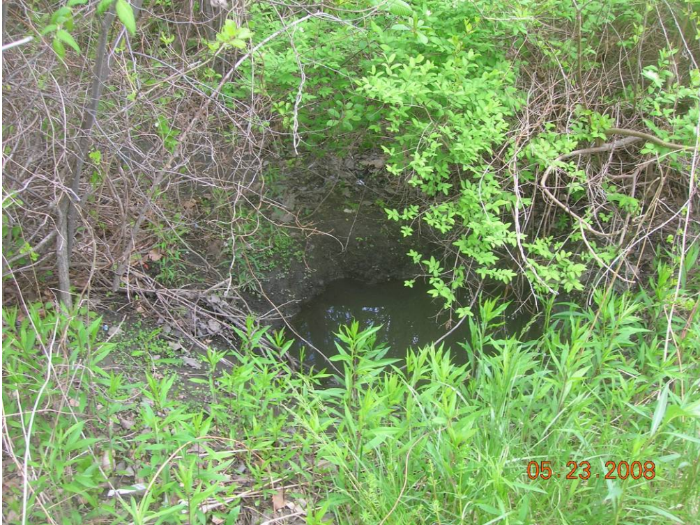
Photo 4 - View of the location of the subsurface outfall pipe identified by EPA between GE Locations 2 and 3.
